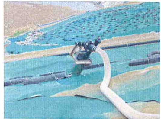
Well head & pipeline for extraction and conveyance of LFG
