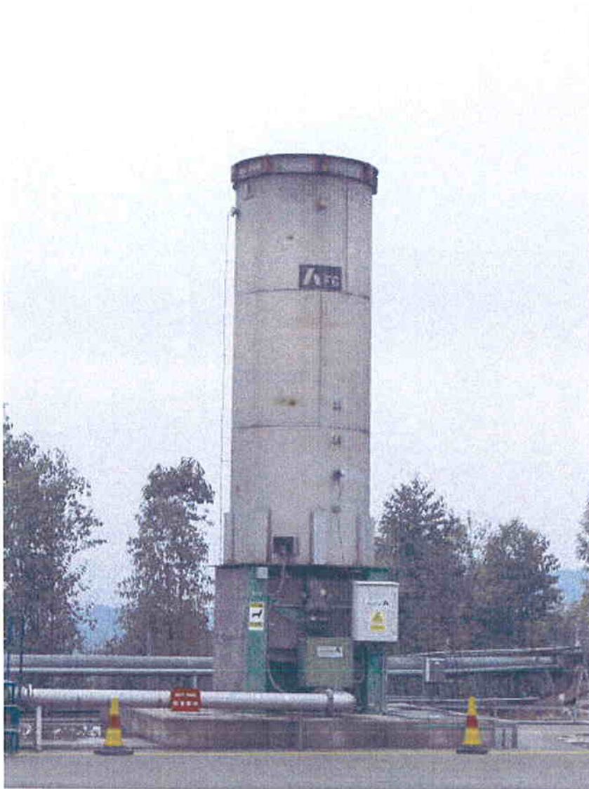
Flare for combustion of LFG
