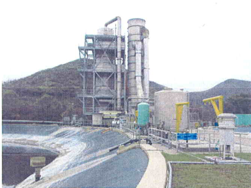
Ammonia stripping plant using LFG to heat up raw leachate
