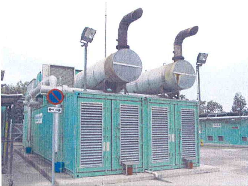
Gensets for power generation using LFG
