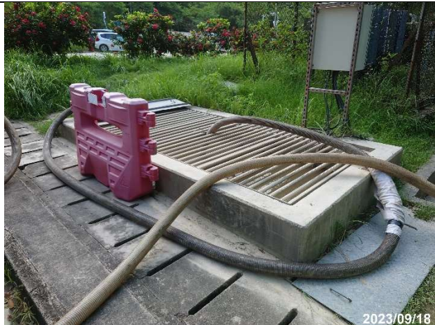
Photo 12-20 Existing Channel near the gate (Runoff from carpark flow to the channel.)
