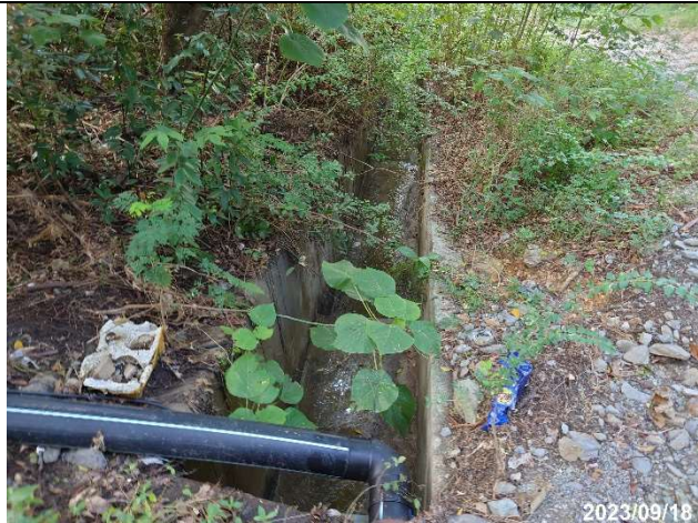
Photo 12-20 Existing Channel near the gate (Runoff from carpark flow to the channel.)
