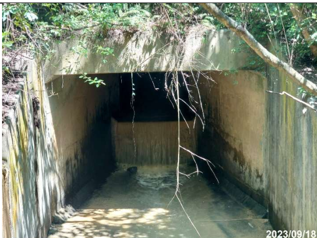
Photo 12-31 Outlet of Box Culvert under Portion C
