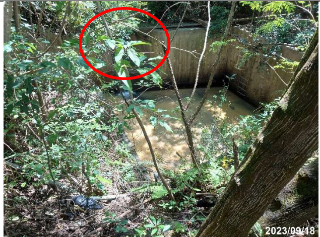
Photo 12-30 Outlet of Box Culvert under Portion C
