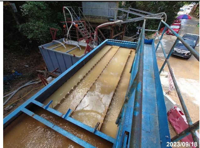
Photo 12-38 Silt Removal Facility at Portion E3-1
