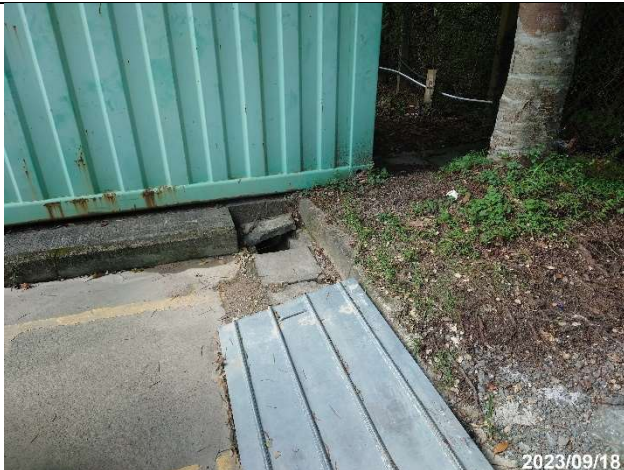
Photo 12-17 Stormwater hole near the gate (Runoff from Car park of NENT Landfill can be flowed directly to the existing channel)
