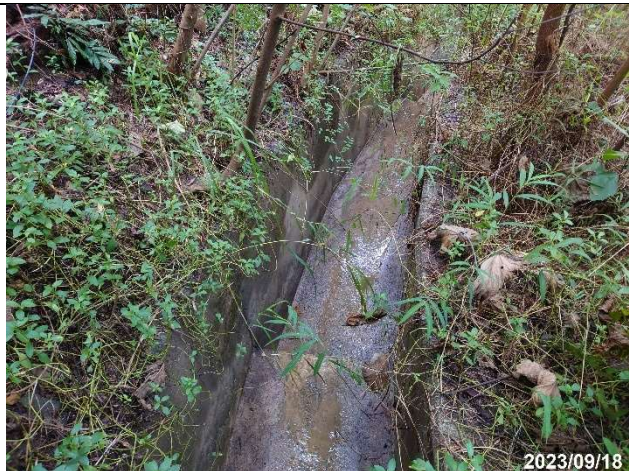
Photo 12-22 Existing channel (Runoff from carpark flow to the channel.)
