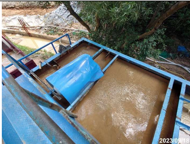
Photo 12-37 Silt Removal Facility at Portion E3-1
