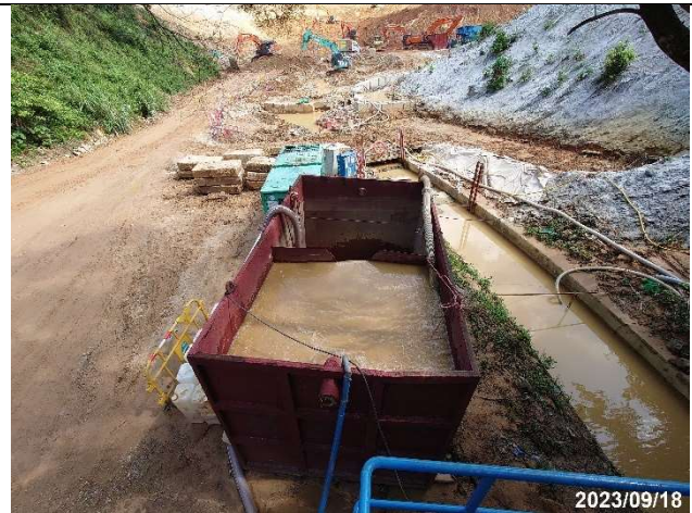
Photo 12-38 Silt Removal Facility at Portion E3-1
