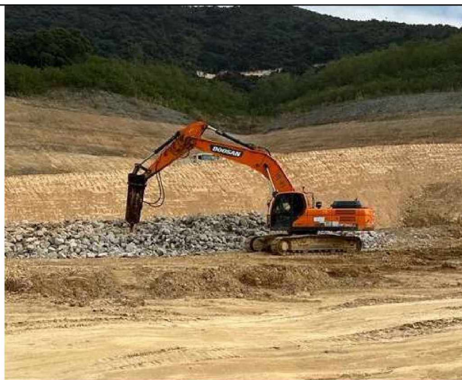
Reminder 2: Water spray or dust suppression chemical shall be provided during mechanical breaking operation in SBA.
