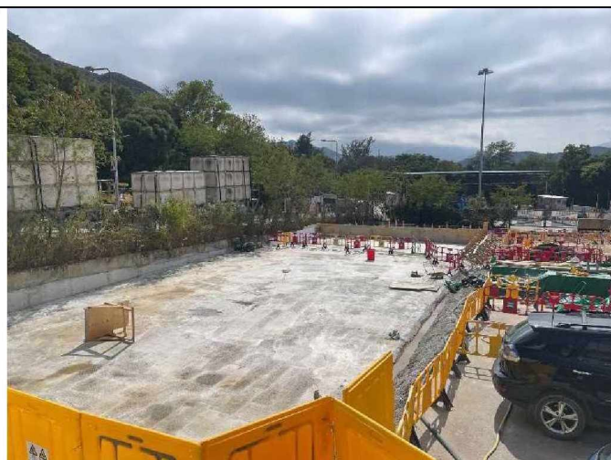
The exposed earth was paved to prevent dust dispersion.
