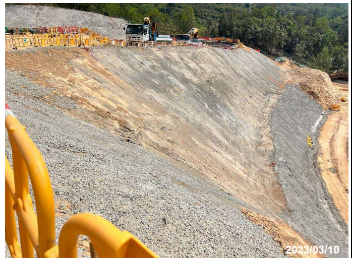
Photo 16 Application of cement slurry at Portion A
