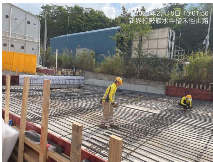
Photo 3 FSB Rebar Fixing at Portion D
