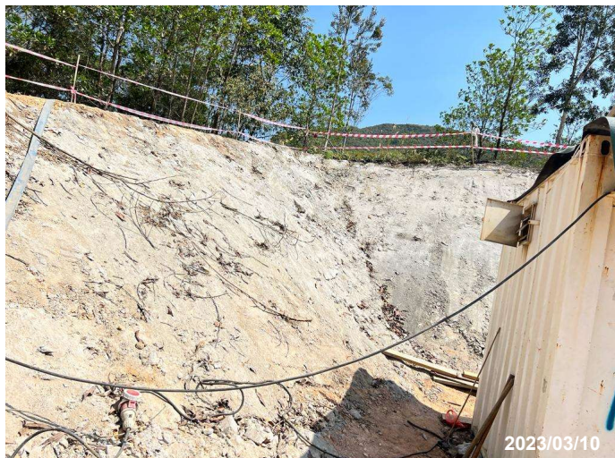
Photo 15 Application of cement slurry at Portion A
