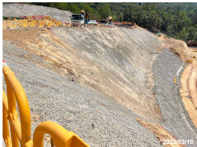
Photo 19 Hydroseeding at bare slope at Portion E3-2
