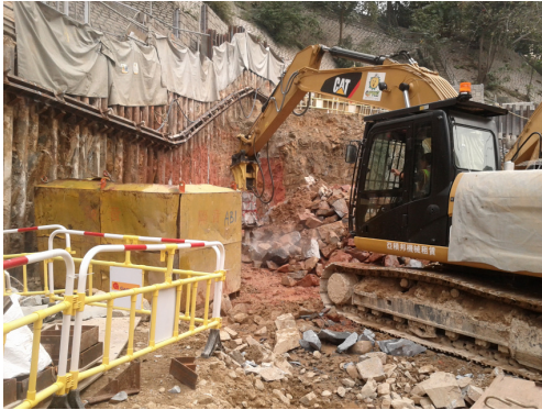
Figure 2.2 Adoption of Portable Noise Barrier
