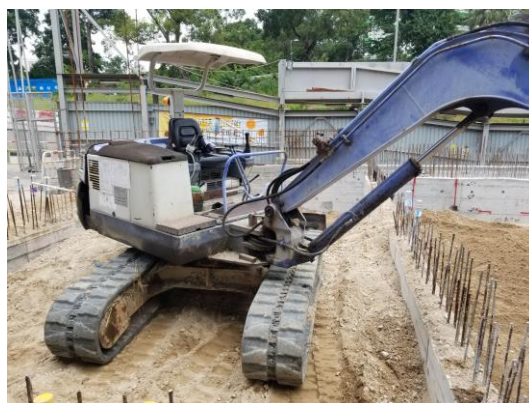
4. Construction works to on-grade slab
