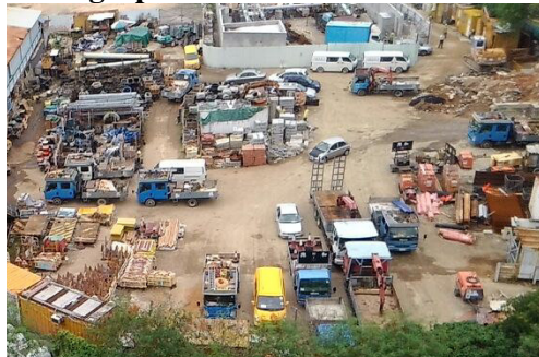
(Photo 1: Construction works conducting outside KTD Project Area.)
