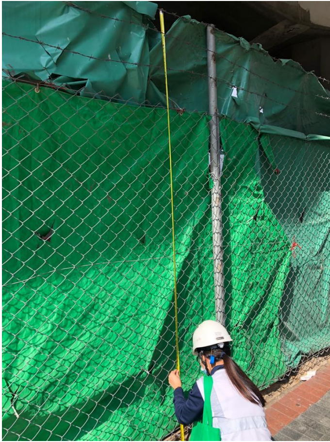
Figure A3 Hoarding along the site boundary
