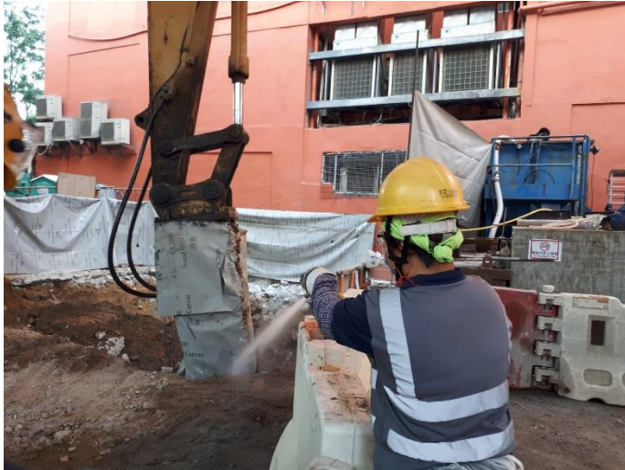
Figure A1 Noise barrier mat fully covered for the breaker's head and water spraying during breaking
