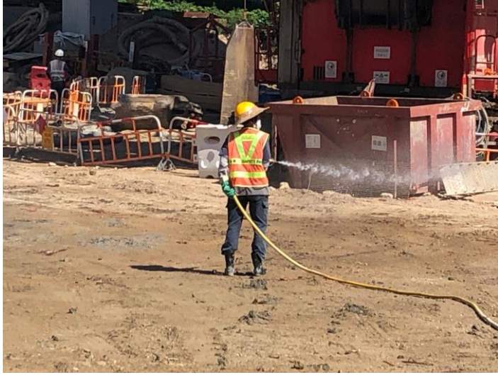
Figure A1 Water spraying
