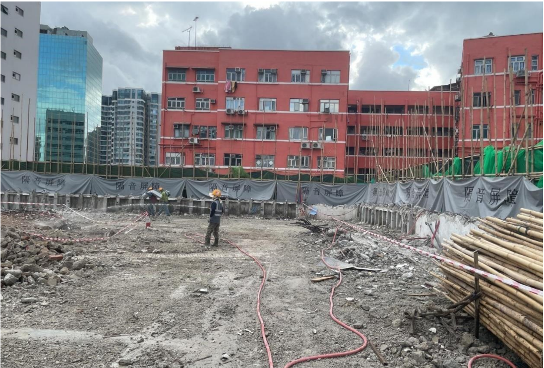
Figure A1: Properly erected noise barrier mat surrounding 4 sides of the building
