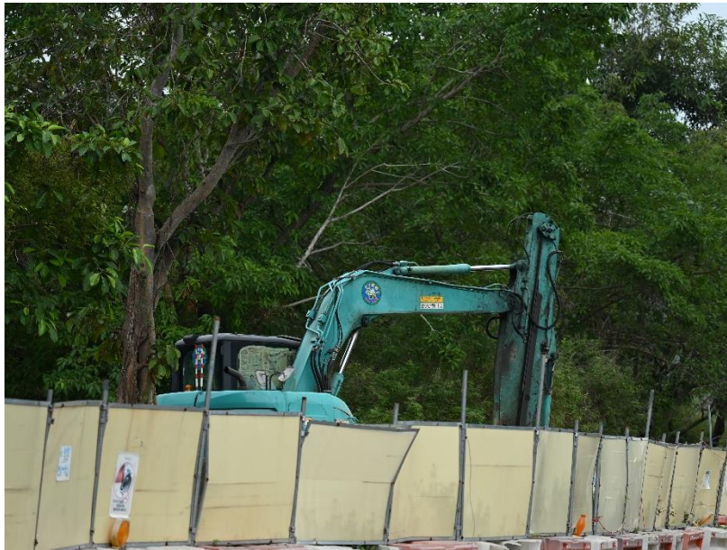
Excavation (Non-project-related, taken on 23 November 2024)
