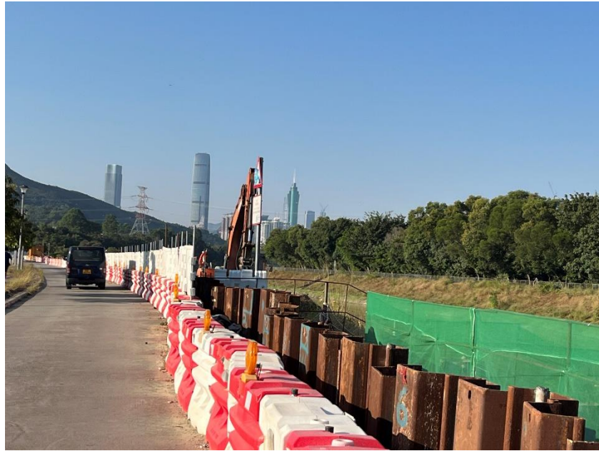
Sheet-piling (Non-project-related, taken on 07 November 2024)
