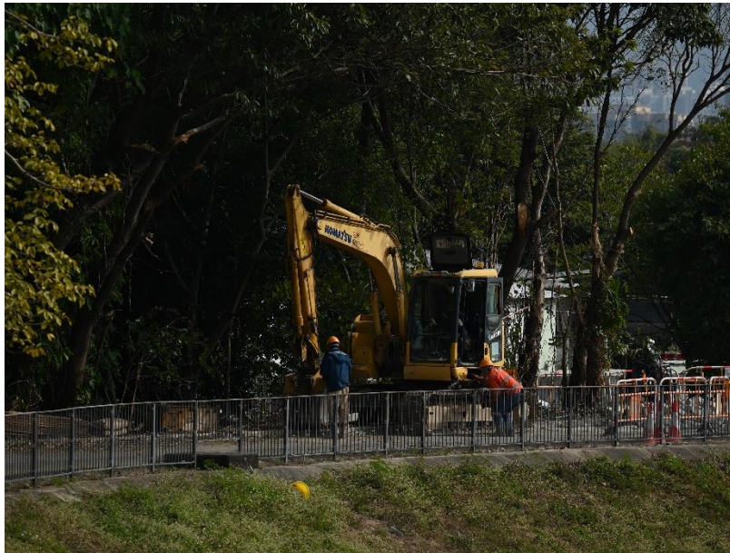
Excavation (Non-project-related, taken on 24 December 2024)
