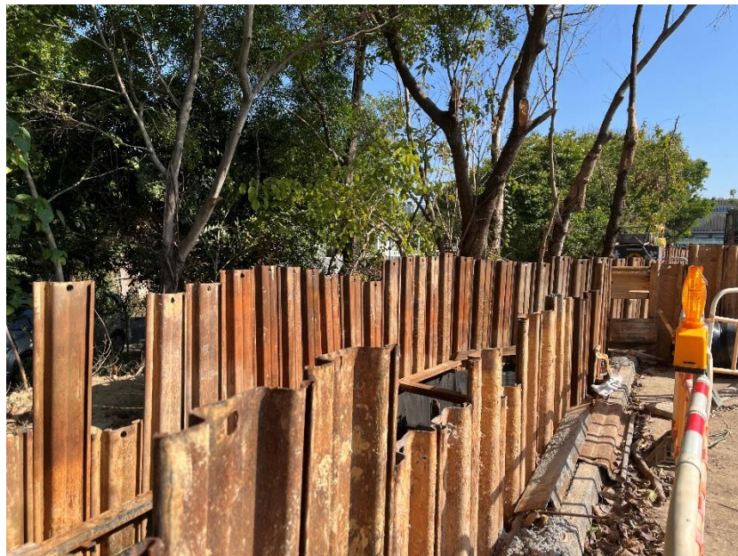
Sheet-piling (Non-project-related, taken on 28 January 2025)
