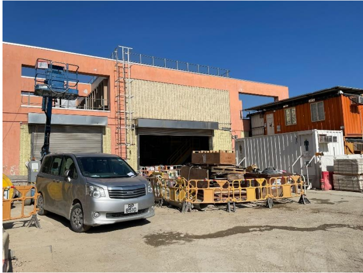
DE/2018/04 –Compressor House
