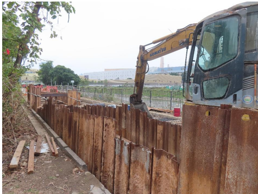
Sheet-piling (Non-project-related, taken on 14 February 2025)
