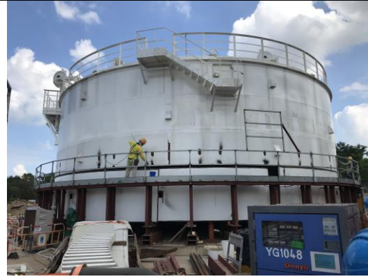
Bio Gas Tank
