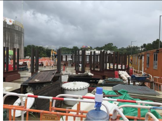
Bio Gas Tank
