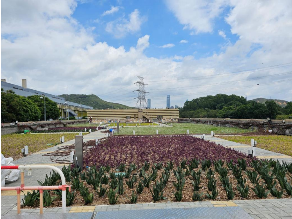
General View of HCF Roof
