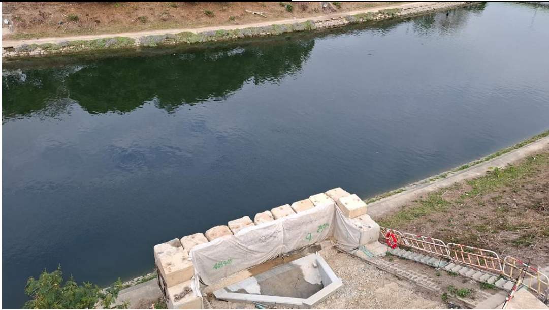
Commencement of Outfall Construction
