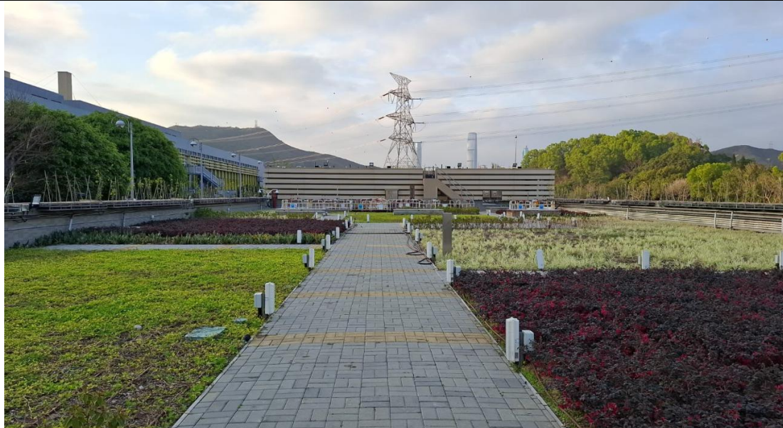
General view of HCF Roof Landscape Softworks
