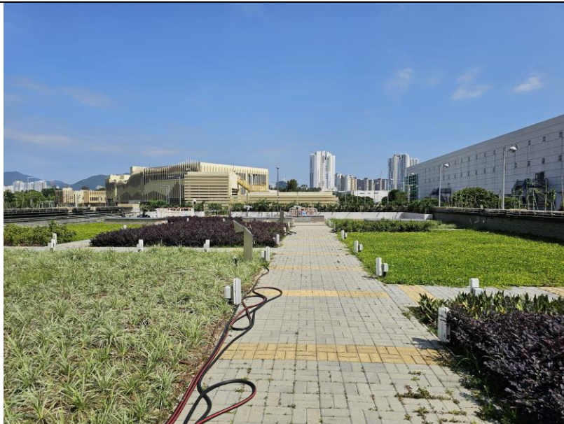
General view of HCF Roof Landscape Softworks
