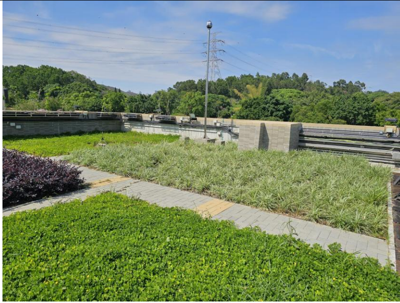
General view of HCF Roof Landscape Softworks
