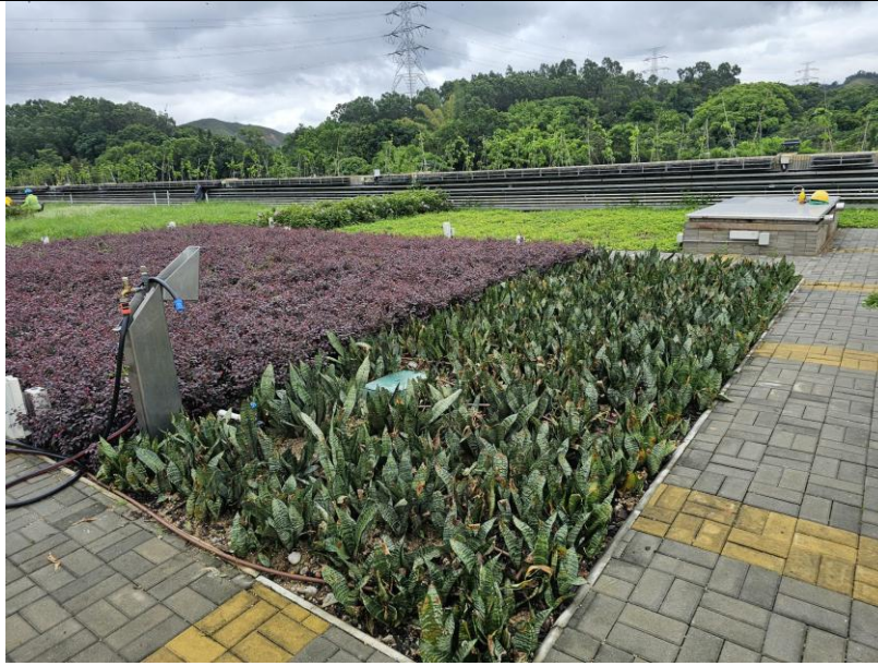
General view of HCF Roof Landscape Softworks
