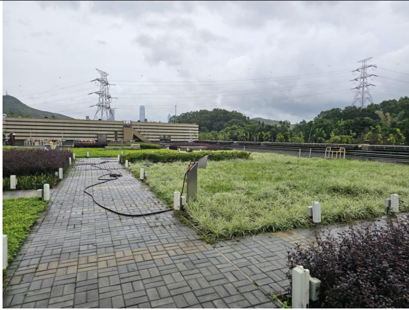
General view of HCF Roof Landscape Softworks
