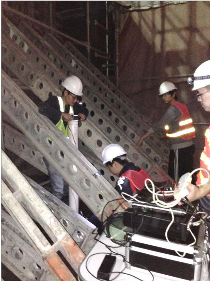
Figure 4.6 Hammer Impact Test at Pt1
