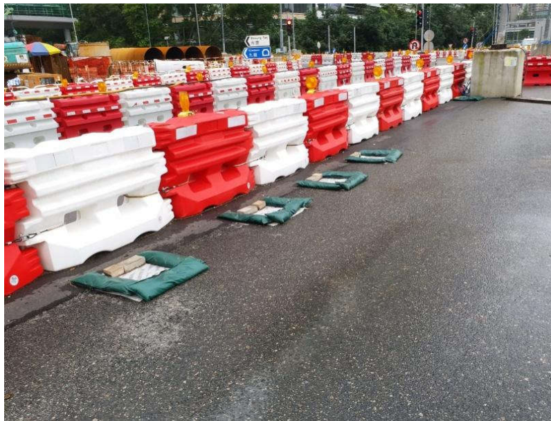
Gully were protected and covered by geotextile.
