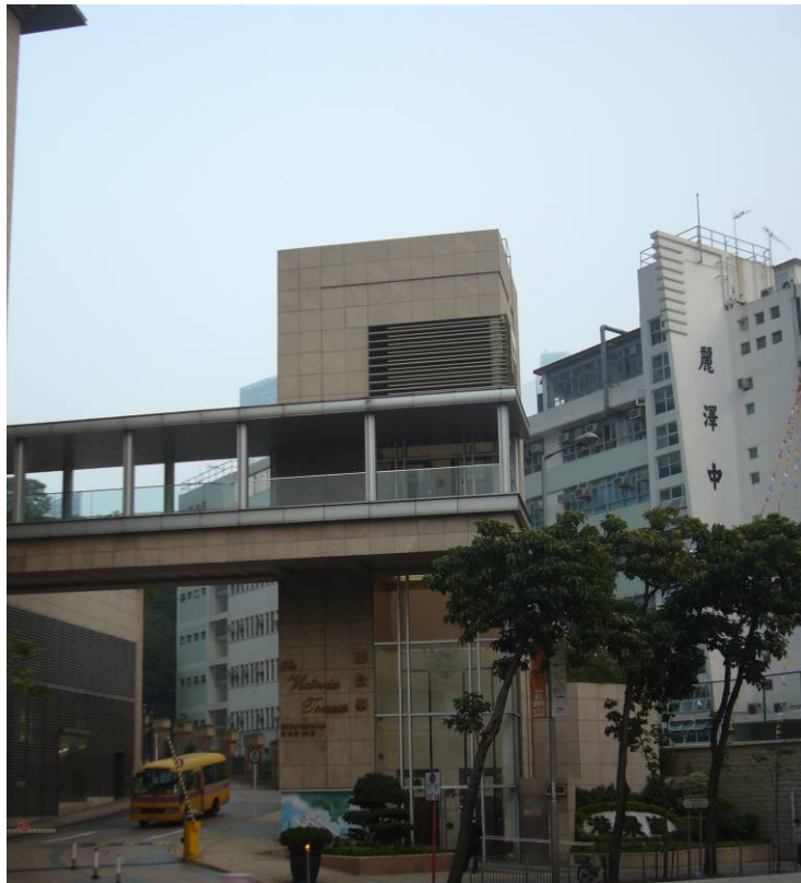
Alternative location of AM 17 and CN 34 – Roof of Lift Building, The Victoria Towers
