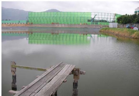
Plate 5 Construction Activities at Point Count Location MPV-1/P9 for Wo Shang Wai Development Project
