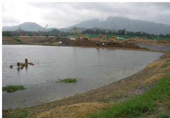
Plate 6 Excavation Works at Point Count Location MPV-1/P9 for Wo Shang Wai Development Project
