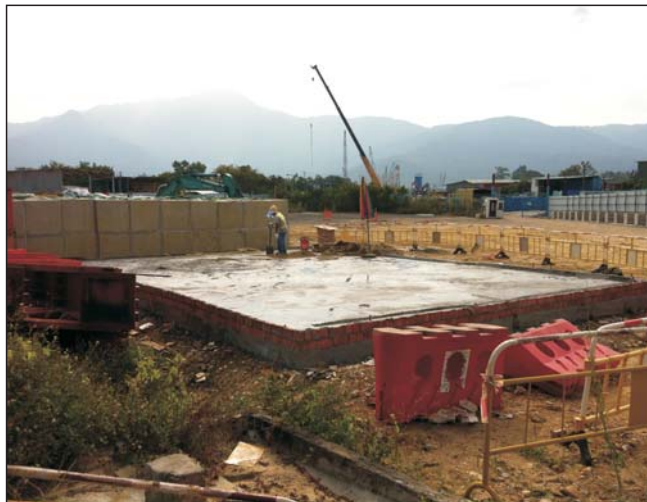
Photo 8: Construction of the base of the biopile
