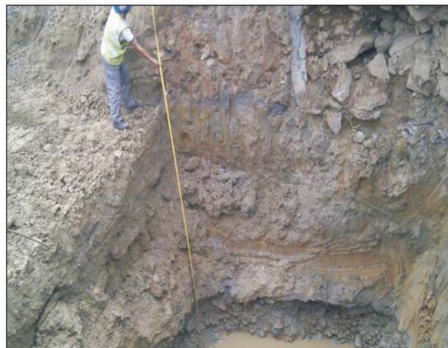
Photo 5: Confirmation of excavation depth
