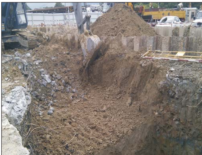
Photo 4: Excavation work at Q-05 after delineation sampling
