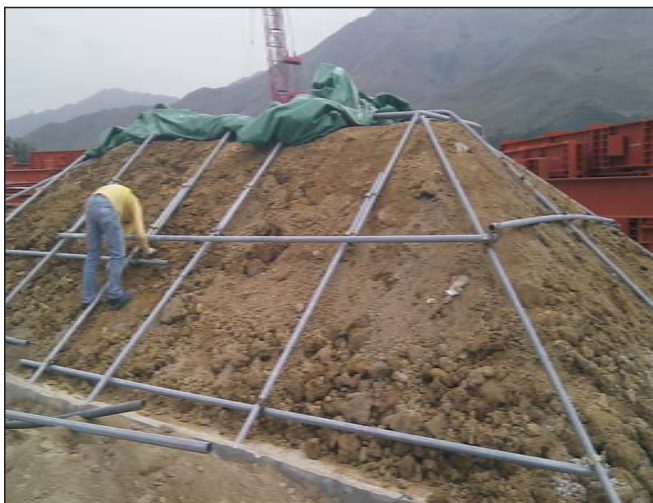
Photo 10: Construction of reinforcing framework for the biopile
