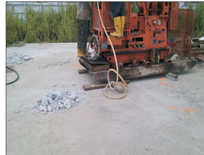
Photo 3: Delineation sampling by rotary drilling at Q-05
