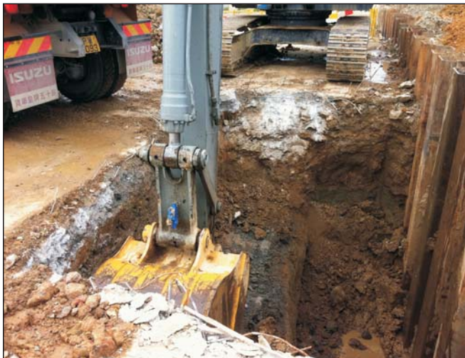
Photo 1: Excavation Work with the use of mechanical machinery at Q-04
