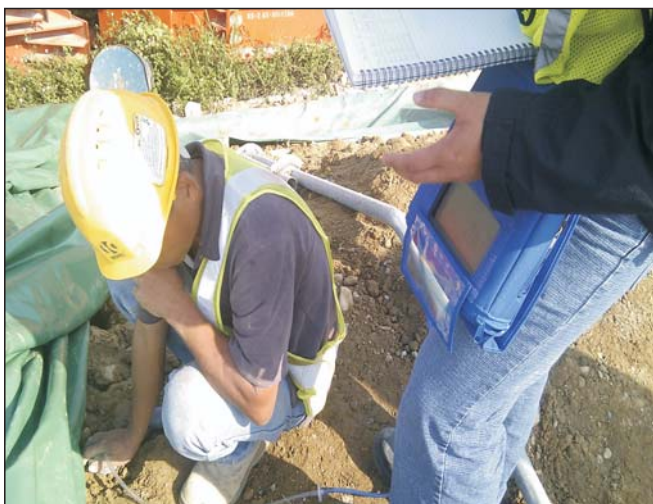
Photo 16: Gas monitoring work during the biopile cleanup progress monitoring
