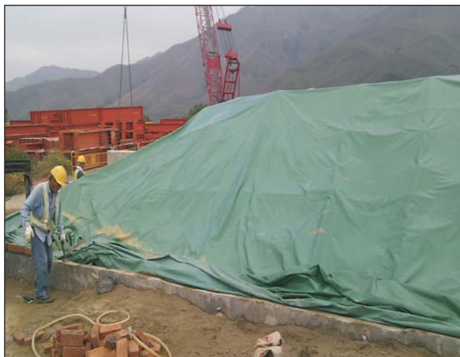
Photo 11: Biopile covered with tarpaulin sheeting
