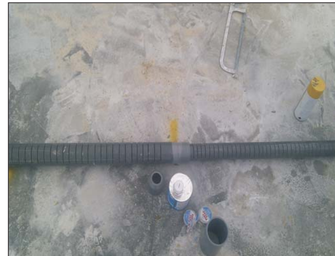
Photo 9: Aeration piping placed at the bottom of the biopile.
