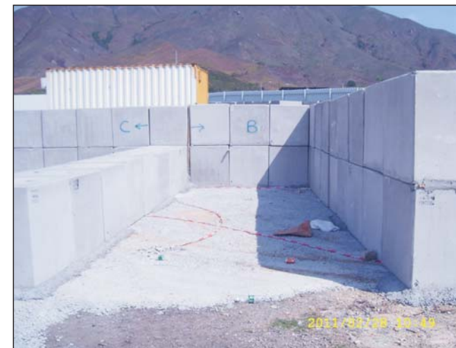
Photo 6: Construction of concrete bunding for temporary storage of contaminated soil
