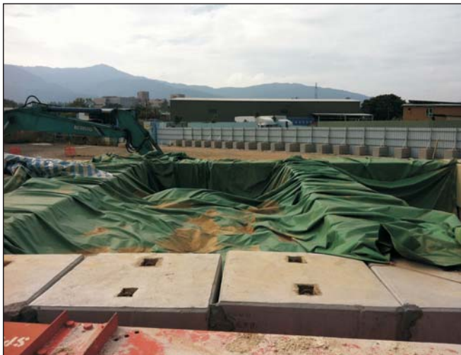
Photo 7: Concrete bunding structure for temporary storage of contaminated soil
