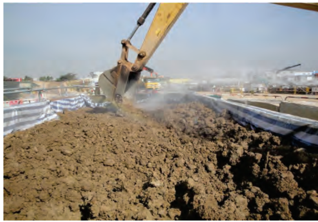
Photo 5: Soil turning with water spray to maintain moisture level of the soil.
