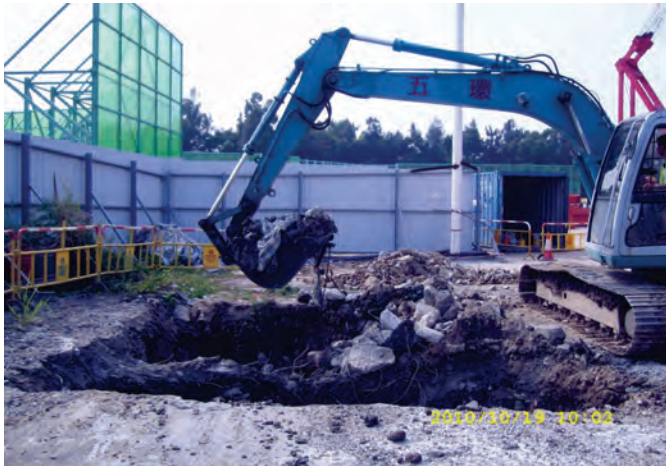
Photo 1: Excavation Work with the use of mechanical machinery at E02
