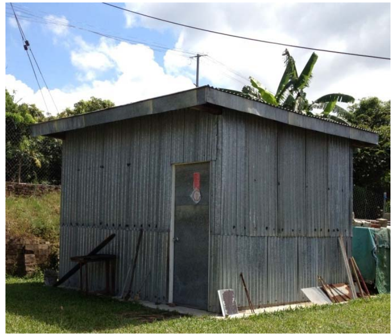
Figure 2D - Photo of store room
