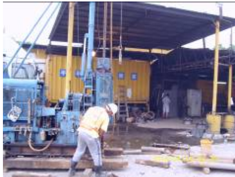
Drilling at sampling location D-02.
