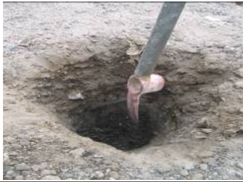
Digging of inspection pits before drilling.
