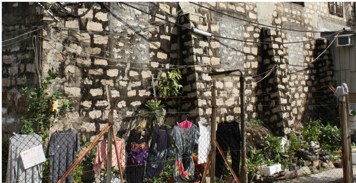
View of the Buttresses on the Southwest Wall of HB-05
