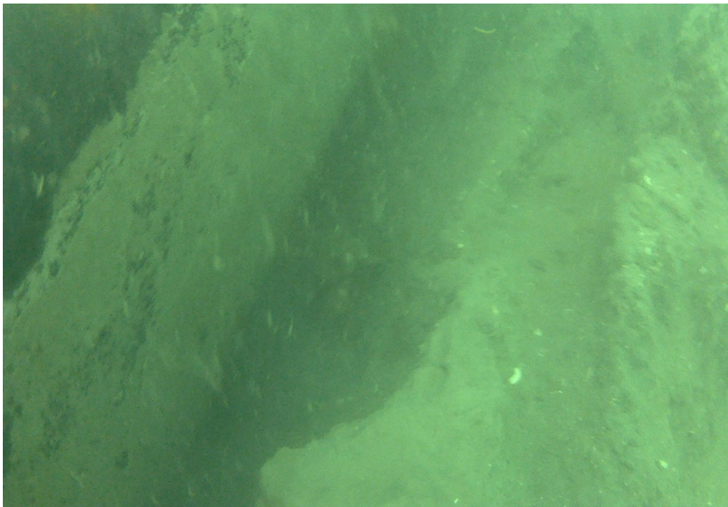
Fig. 10 Geotextile Condition of Silt Curtains
