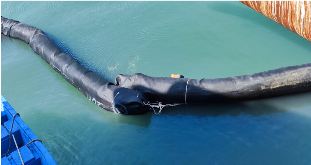
Fig. 2 Connections between Two Adjacent Silt Curtains
