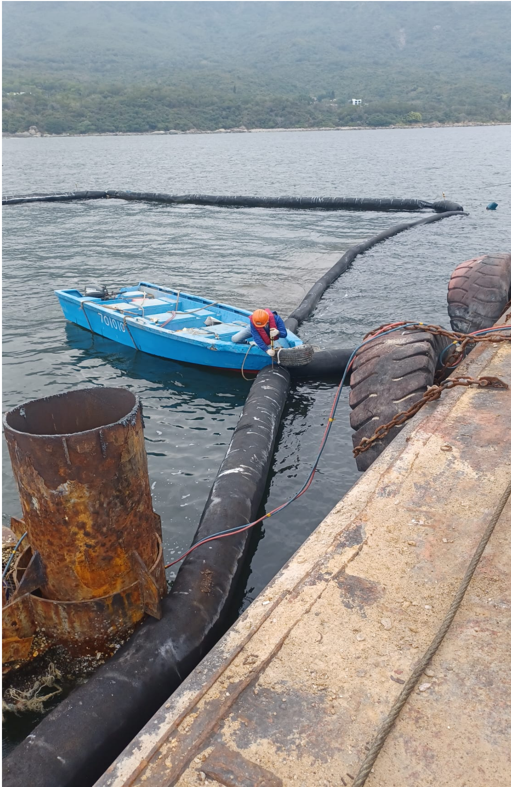
Fig. 9 Connections between Two Adjacent Silt Curtains
