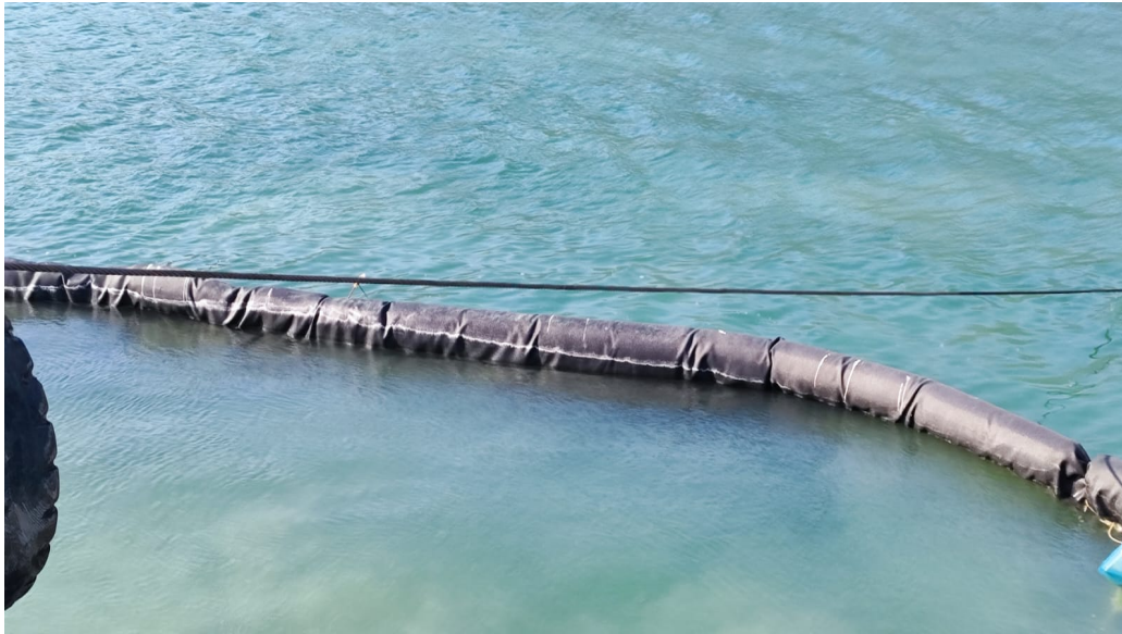
Fig.4 Connections between Two Adjacent Silt Curtains
