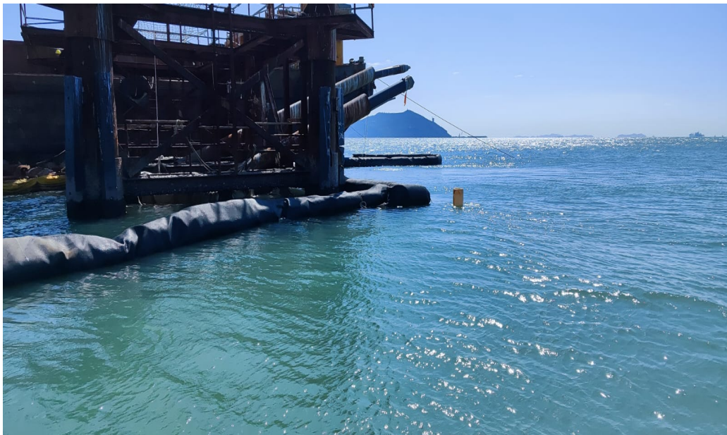
Fig. 1 Silt Curtain Laying Condition
