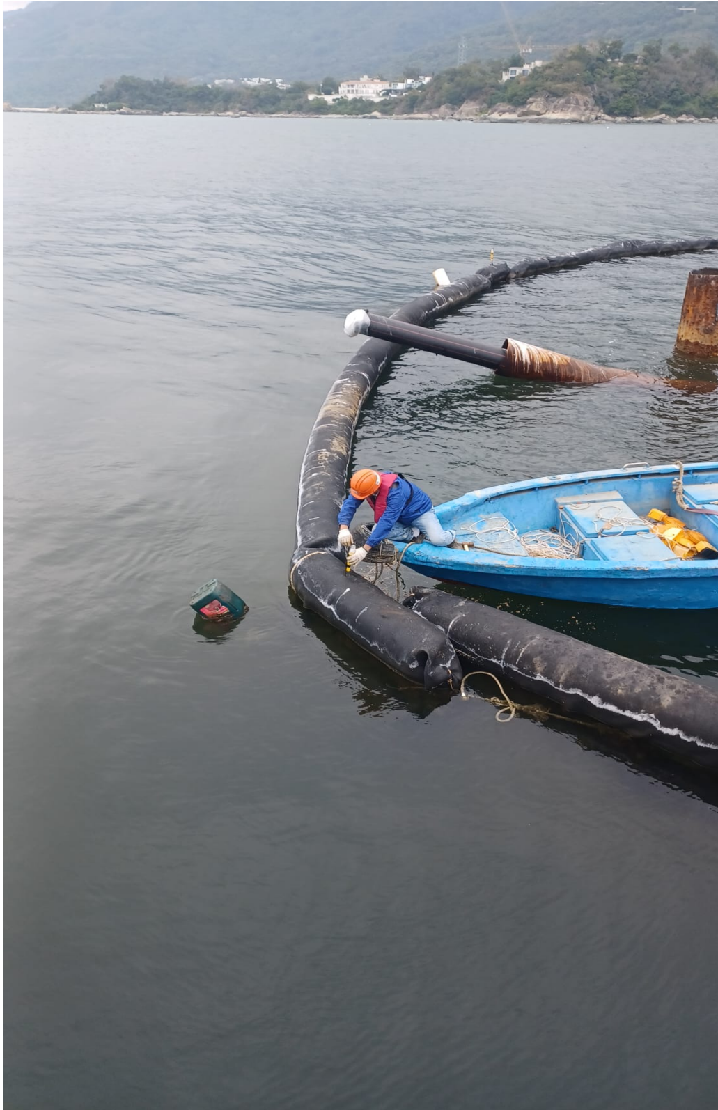
Fig. 7 Connections between Two Adjacent Silt Curtains
