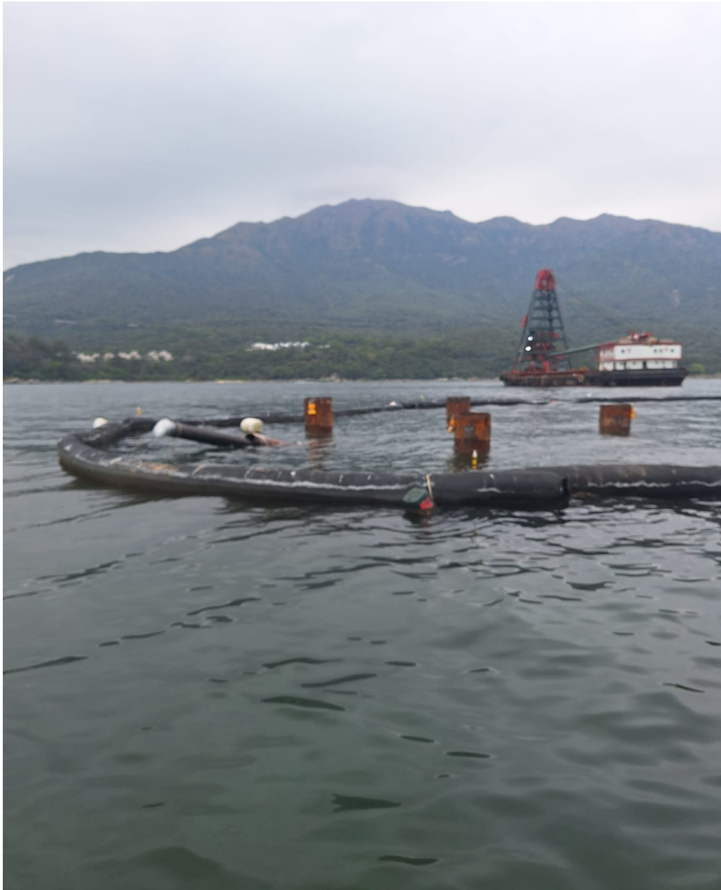
Fig. 5 Connections between Two Adjacent Silt Curtains
