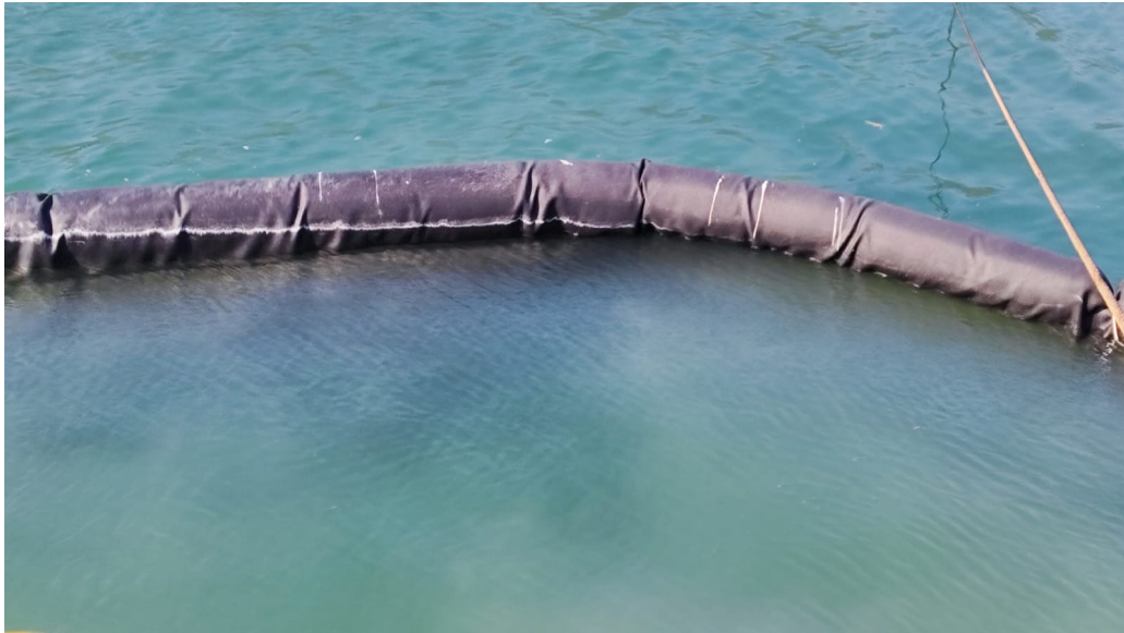
Fig. 6 Connections between Two Adjacent Silt Curtains
