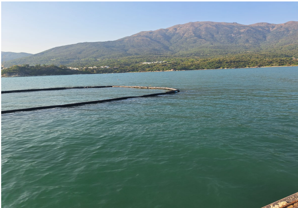
Fig. 1 Silt Curtain Laying Condition
