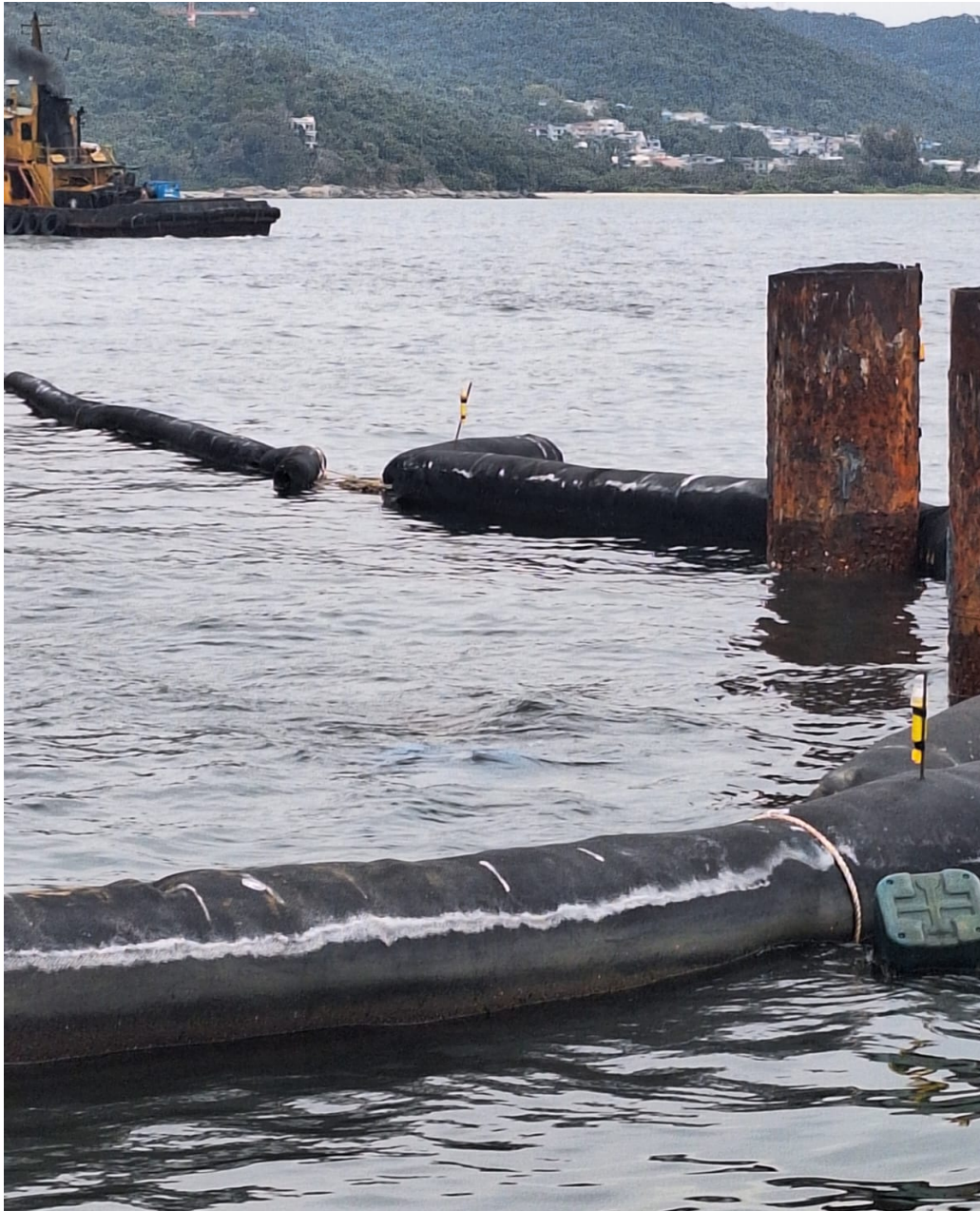
Fig. 6 Connections between Two Adjacent Silt Curtains
