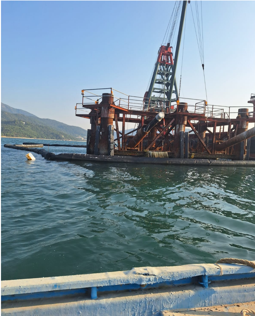
Fig. 2 Connections between Two Adjacent Silt Curtains
