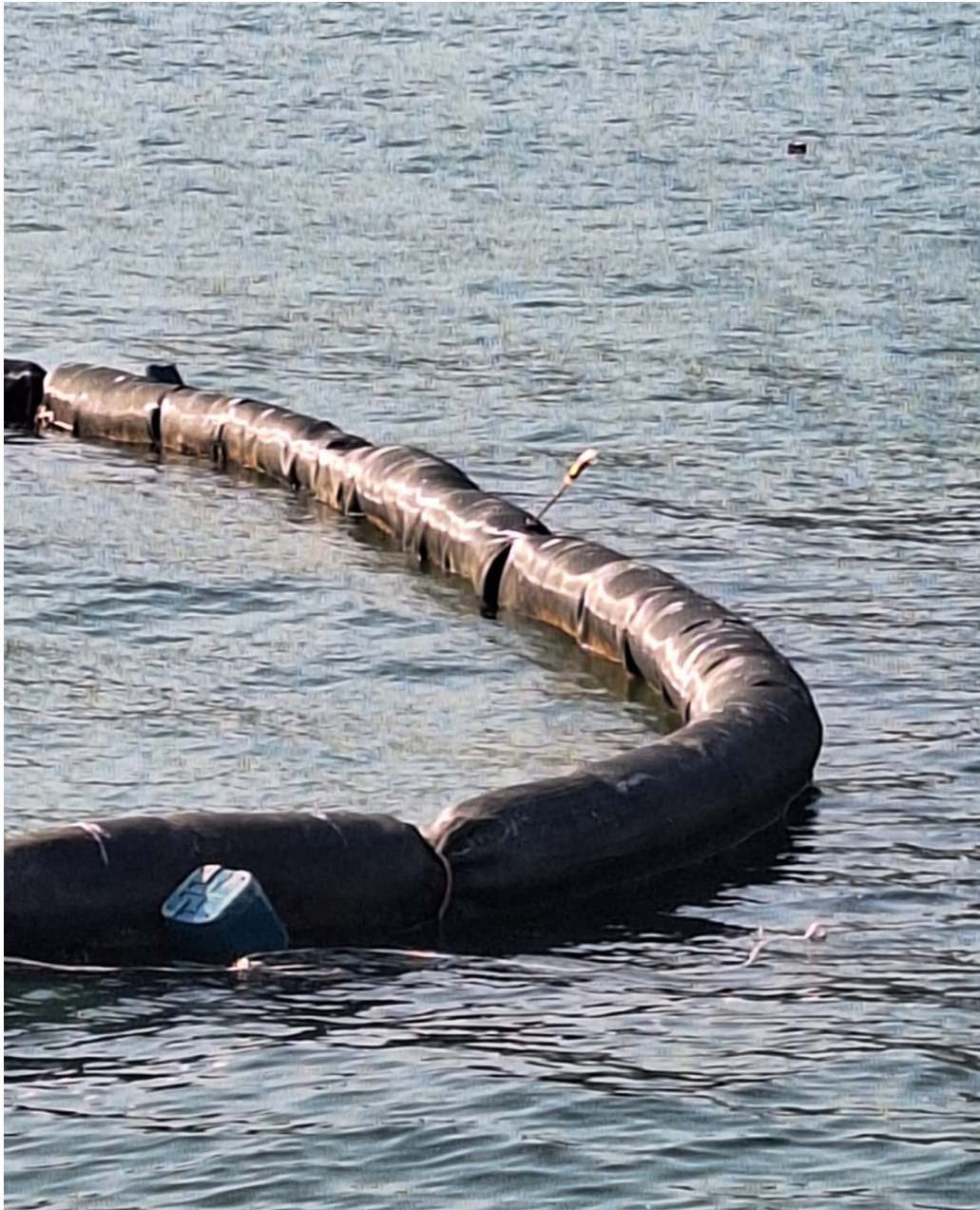
Fig.4 Connections between Two Adjacent Silt Curtains
