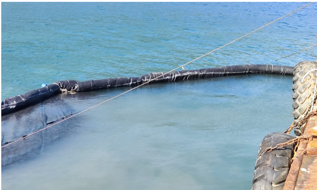
Fig. 5 Connections between Two Adjacent Silt Curtains
