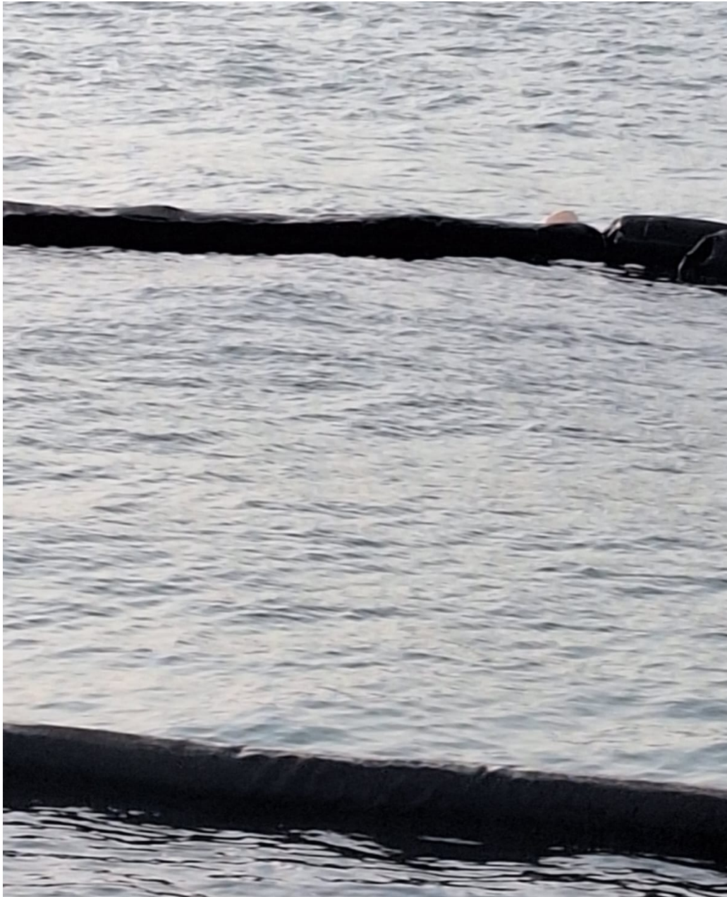
Fig. 2 Connections between Two Adjacent Silt Curtains
