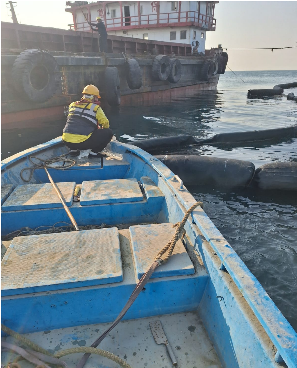
Fig. 6 Connections between Two Adjacent Silt Curtains
