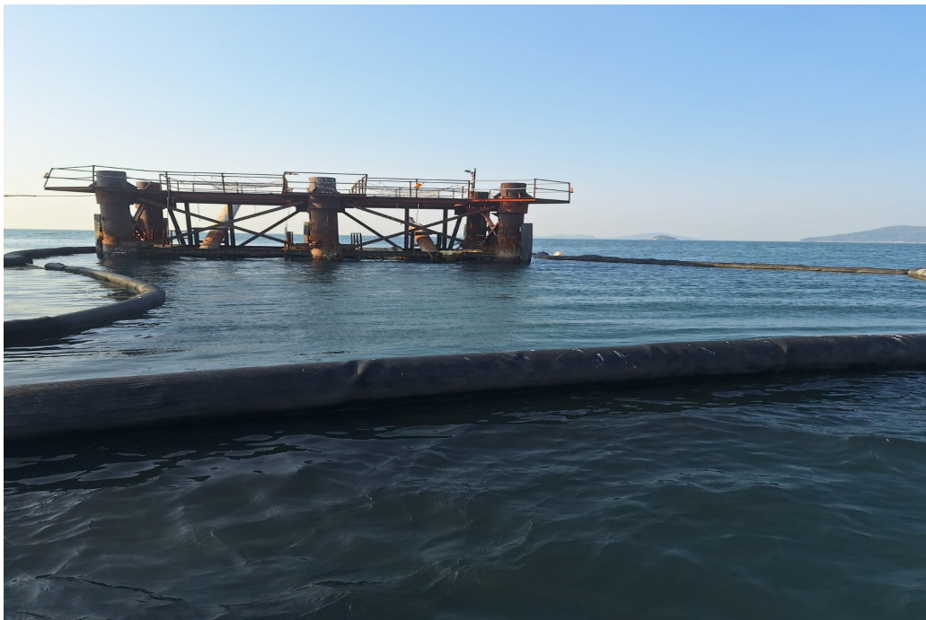
Fig. 1 Silt Curtain Laying Condition
