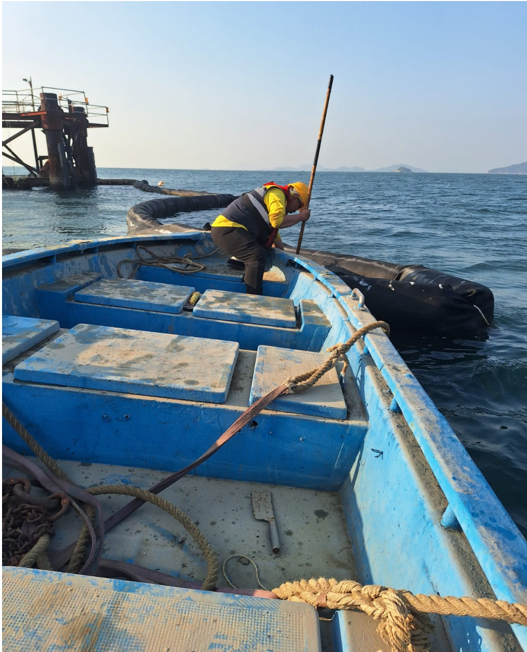
Fig. 5 Connections between Two Adjacent Silt Curtains
