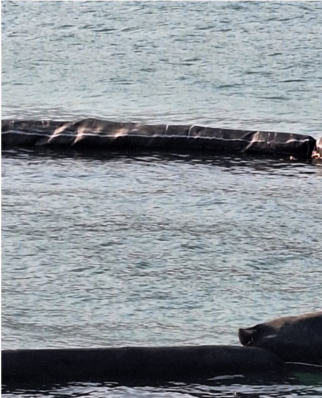
Fig. 3 Connections between Two Adjacent Silt Curtains
