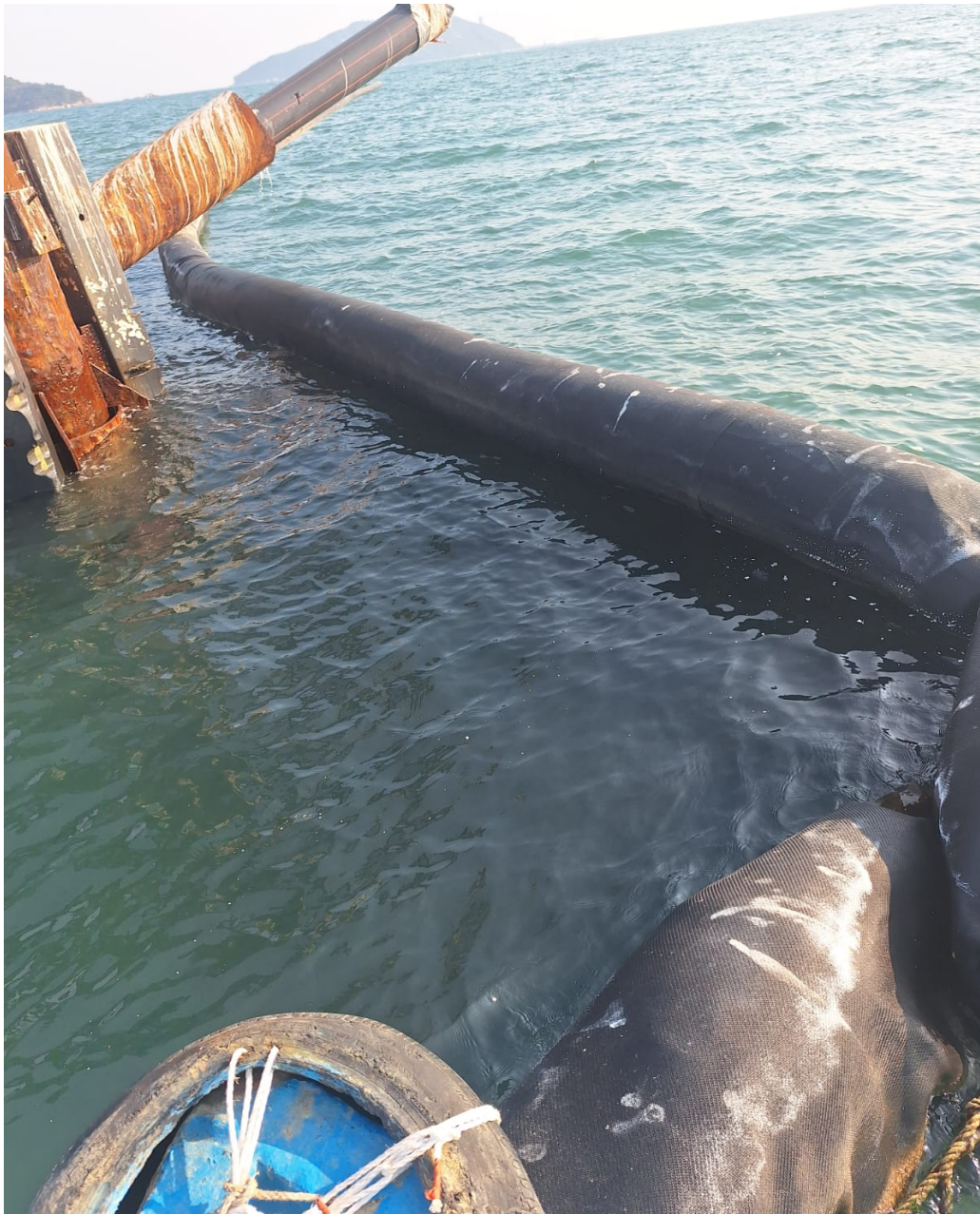
Fig. 8 Connections between Two Adjacent Silt Curtains
