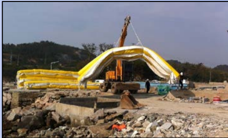
Handling of the silt curtain
