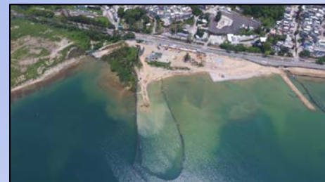
Silt curtain at Lung Mei Beach, May 2018
