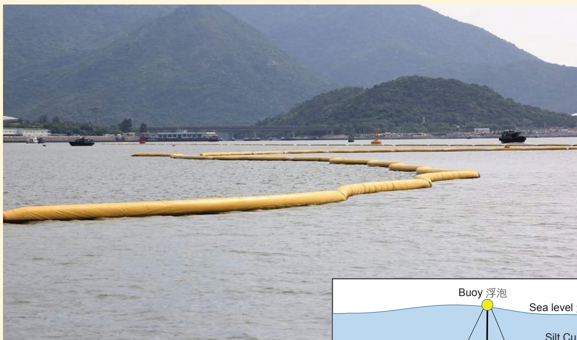
淤泥屏障 Silt curtains
