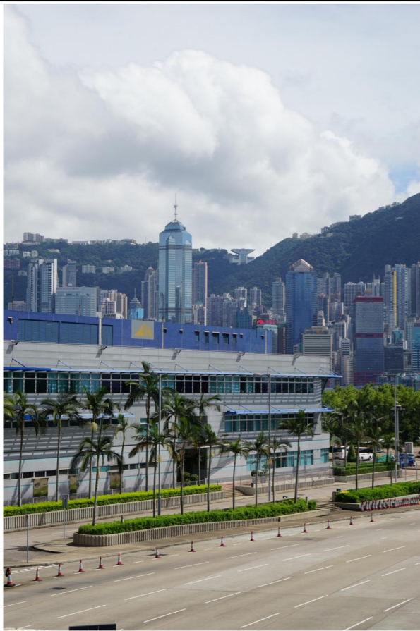
LR2.30 Roadside Plantation next to Western Harbour Tunnel Administration Photo 1 5-8-2014
