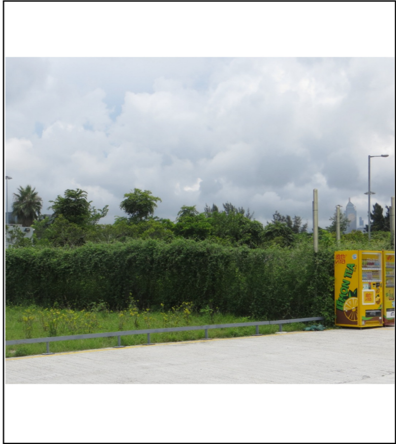
LR2.34 Amenity Planting within Salt Water Pumping Station Photo 2 5-8-2014
