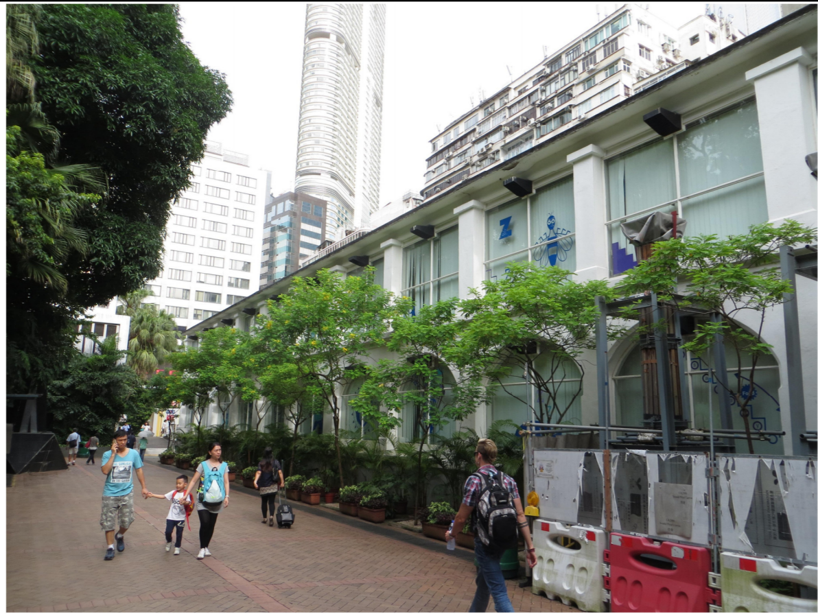
LR4.4 Built Heritage within Kowloon Park Photo 2 - Health Education Exhibition & Resources Centre
