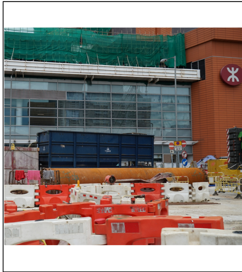
LR2.11 Roadside Plantation along Austin Road Photo 3 6-8-2014
