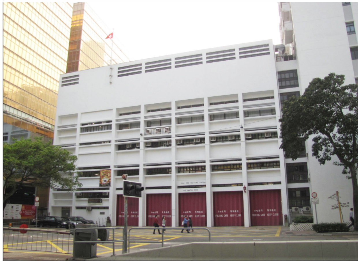
VSR 21 Tsim Sha Tsui Fire Station
