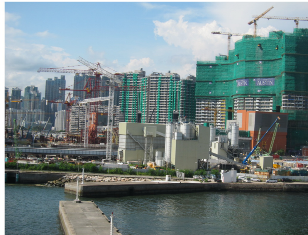
VC04 (LCA02) West Kowloon Cultural District Construction Area
