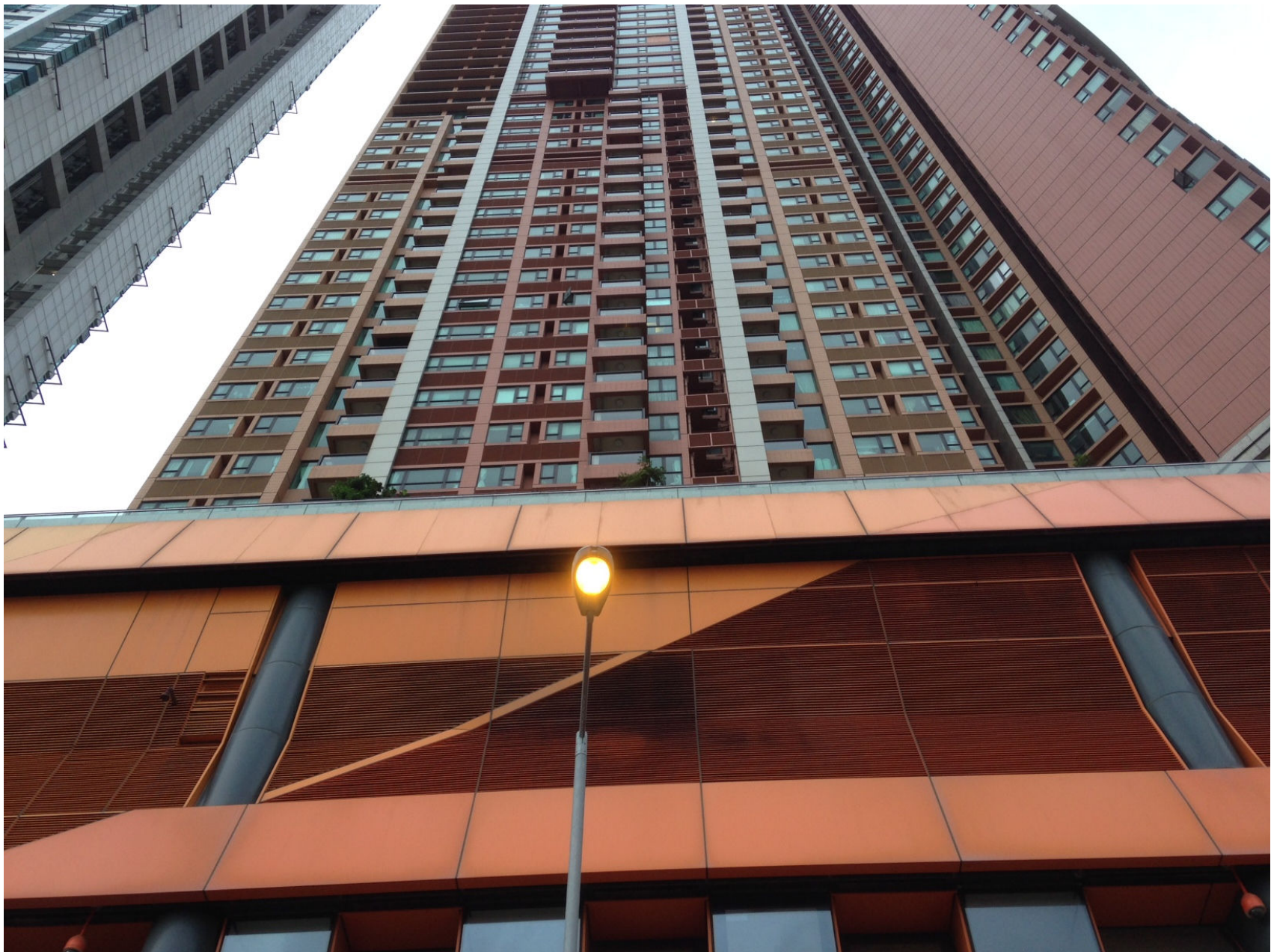
Figure 5) Facade of The Arch facing Austin Road
