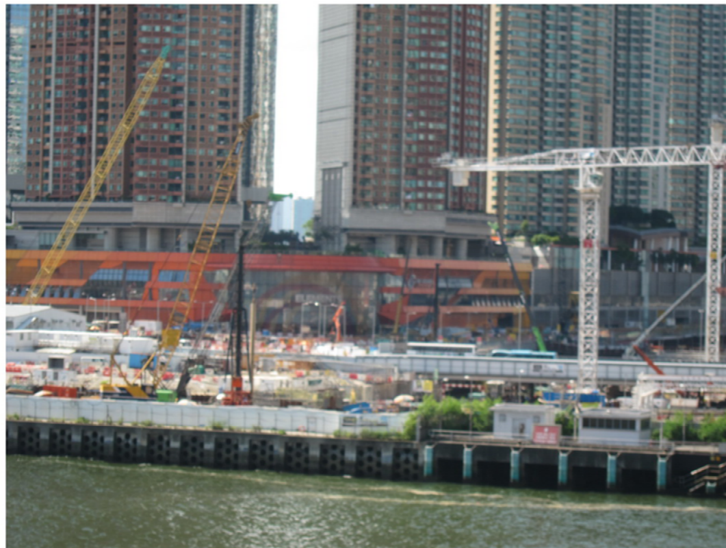
VC03 (LCA02) West Kowloon Cultural District Construction Area
