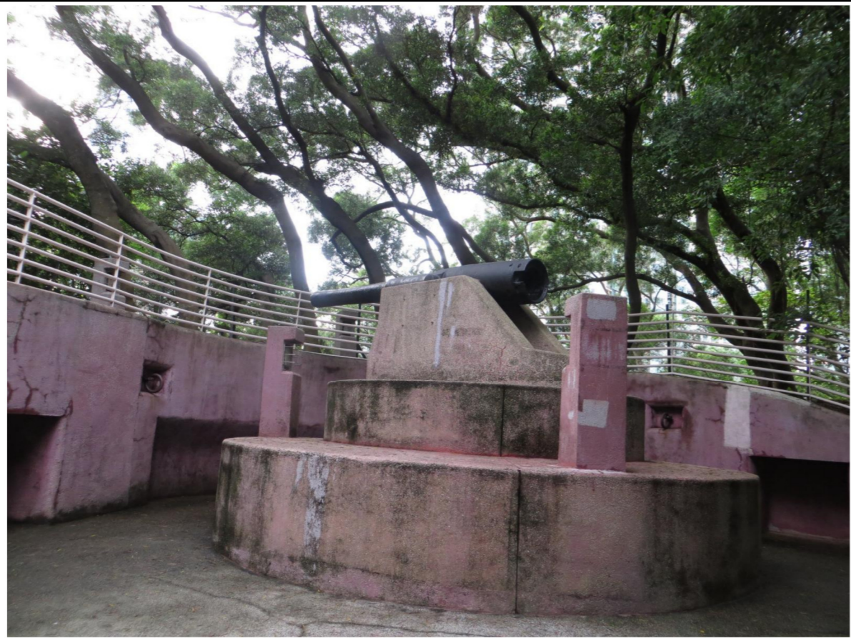
LR4.4 Built Heritage within Kowloon Park Photo 3 - Kowloon West II Battery
