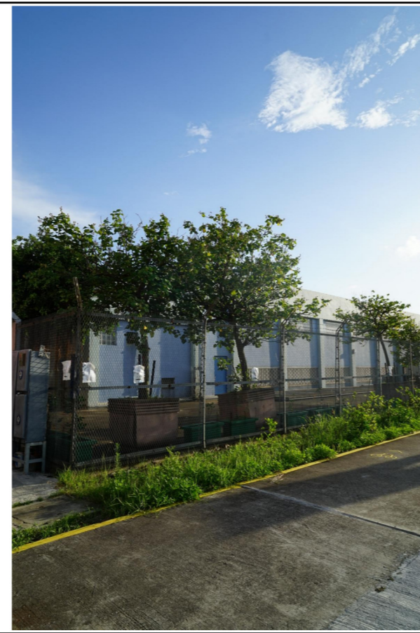
LR2.34 Amenity Planting within Salt Water Pumping Station Photo 1 5-8-2014
