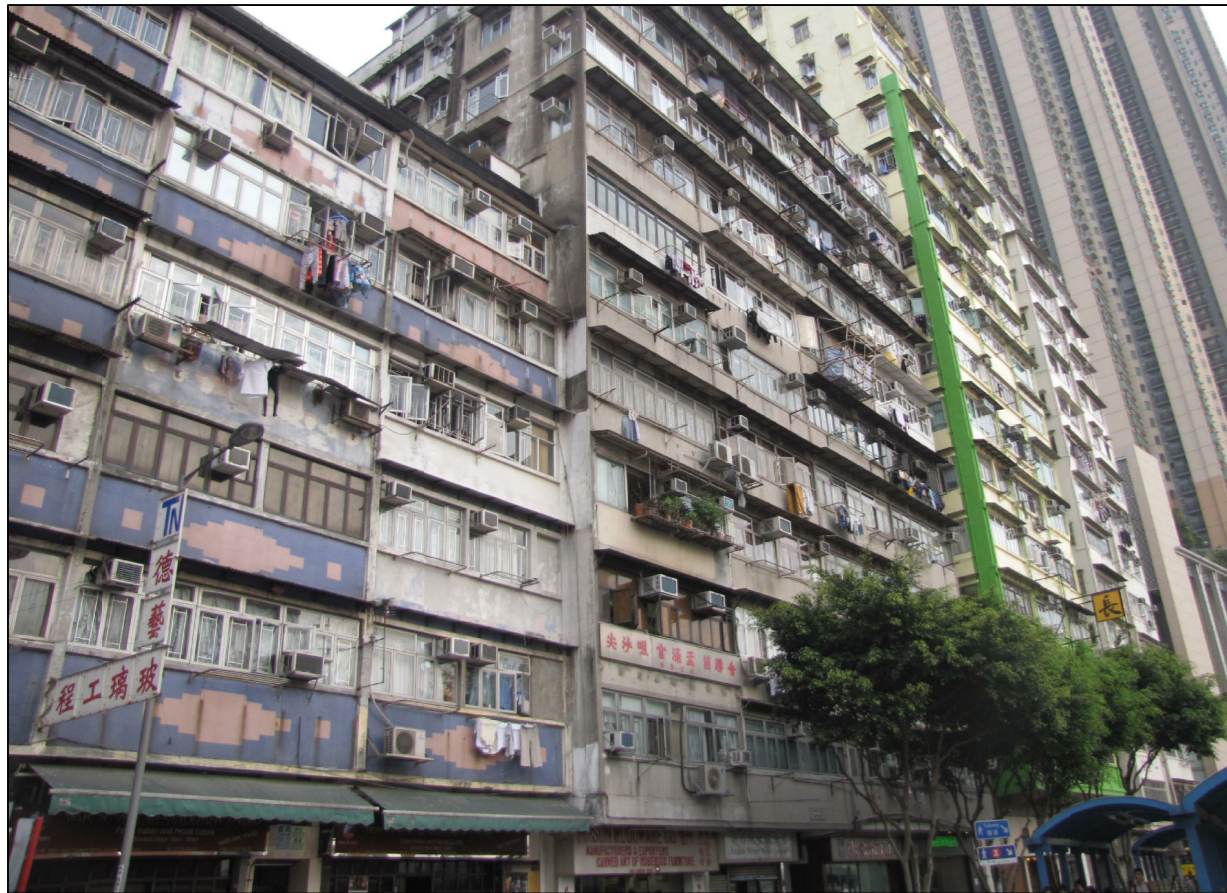
VSR 20 Wai On Building & Wai Hang Building
