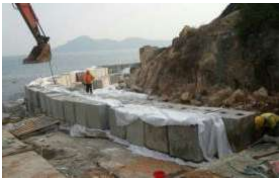
Construction of Working Platform
