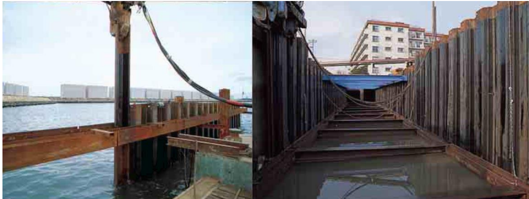
Installation/Extraction of Sheet pile by Vibratory Method
