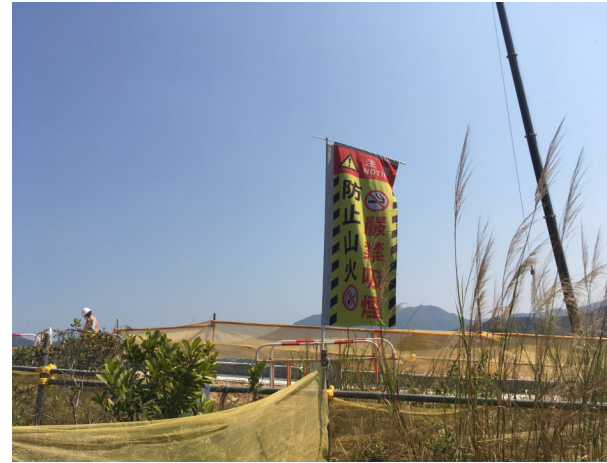
Description: Protective fence properly erected for transplanted Brainea insignis with warning flags.
