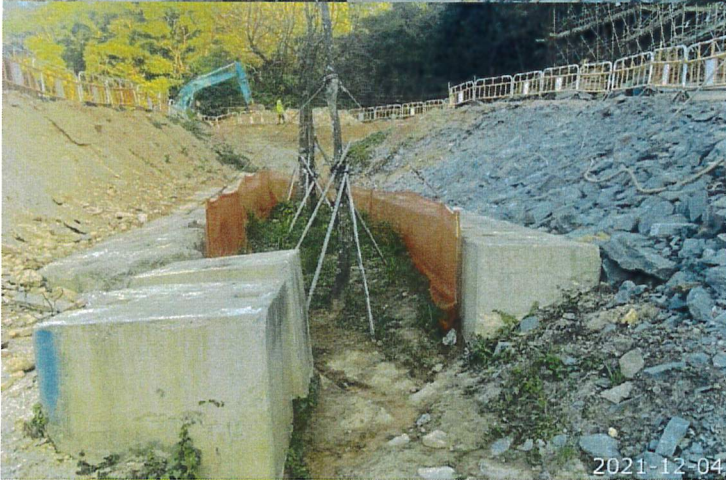
Formation of ditch to guide surface runoff to water pumping location
