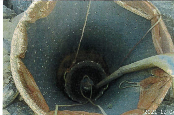
Regular Dewatering at transplanted area
