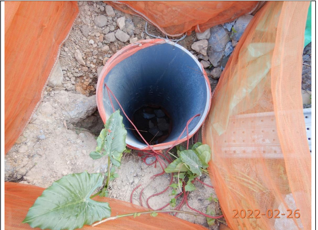
Provision of de-watering well and conduct de-watering during rainy days
