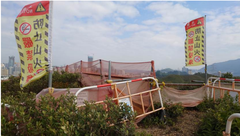
Description: Protective fence for transplanted Brainea insignis are properly erected with warning flags for bushfire prevention.
