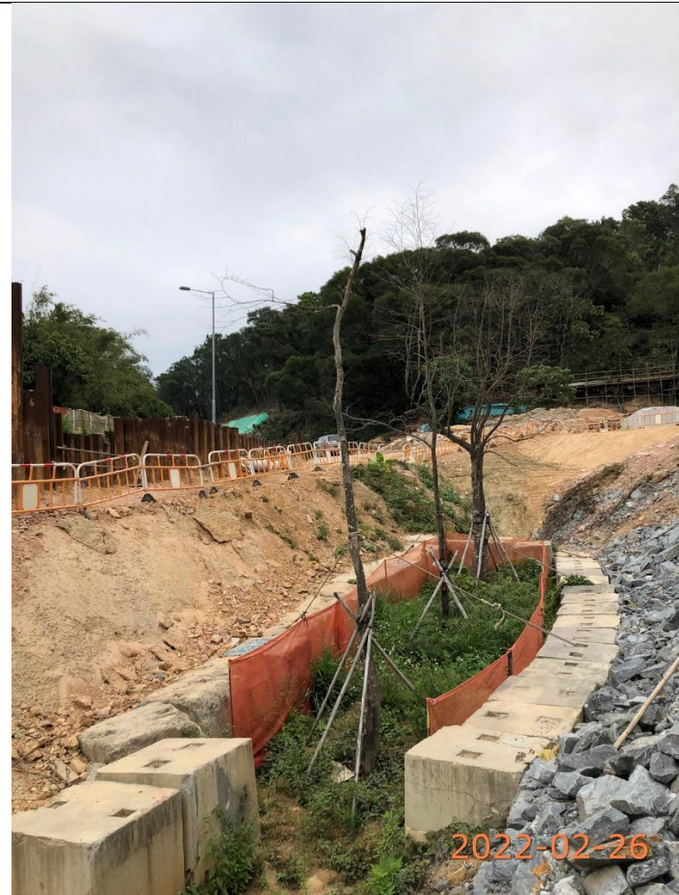
Formation of ditch to guide surface runoff to water pumping location
