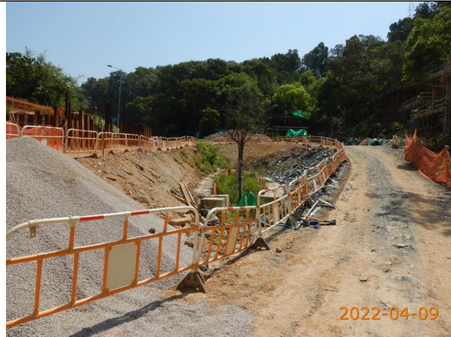
Formation of ditch to guide surface runoff to water pumping location, moist soil surface observed
