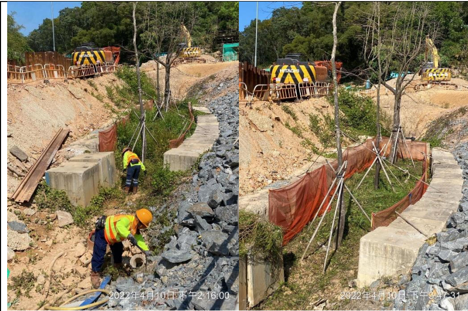
Weeding was carried out on 10 April 2022
