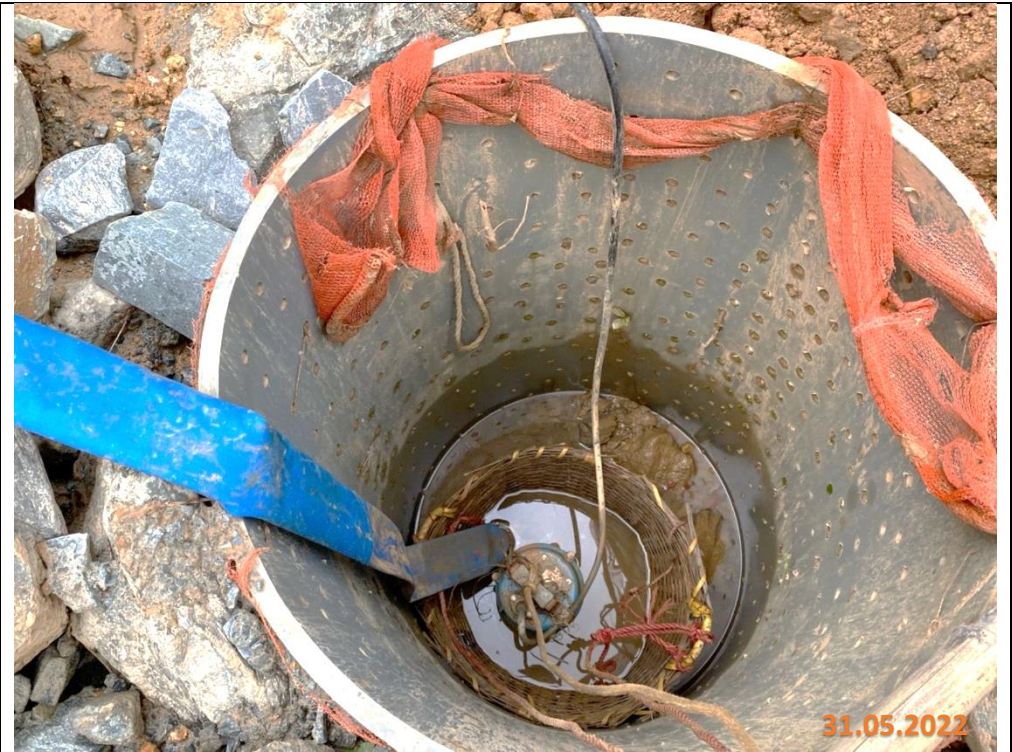
Submersible pump in place and dewatering was carrying out to drain away the collected surface runoff when it was raining
