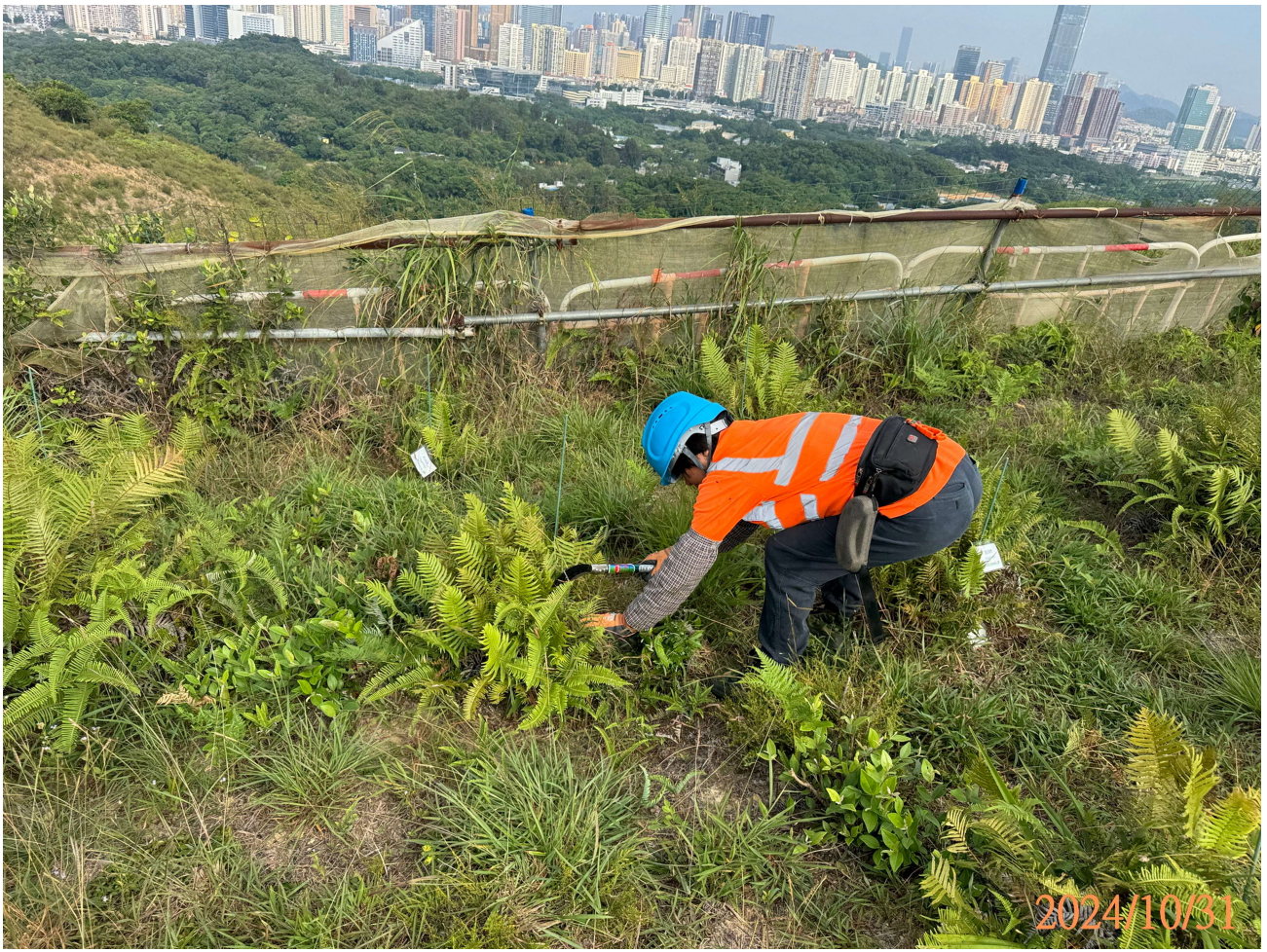
Maintenance works & inspection_3
