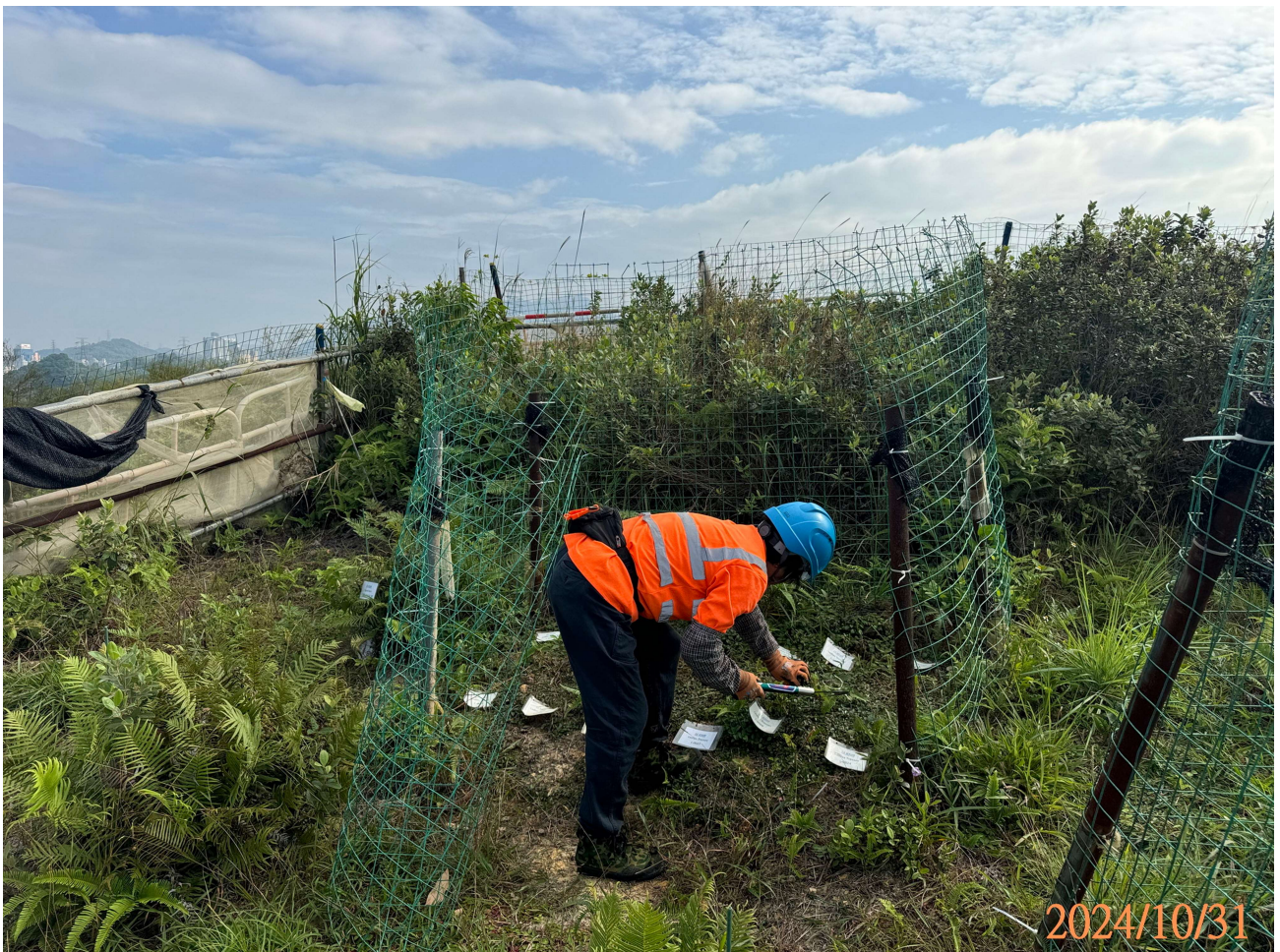
Maintenance works & inspection_4
