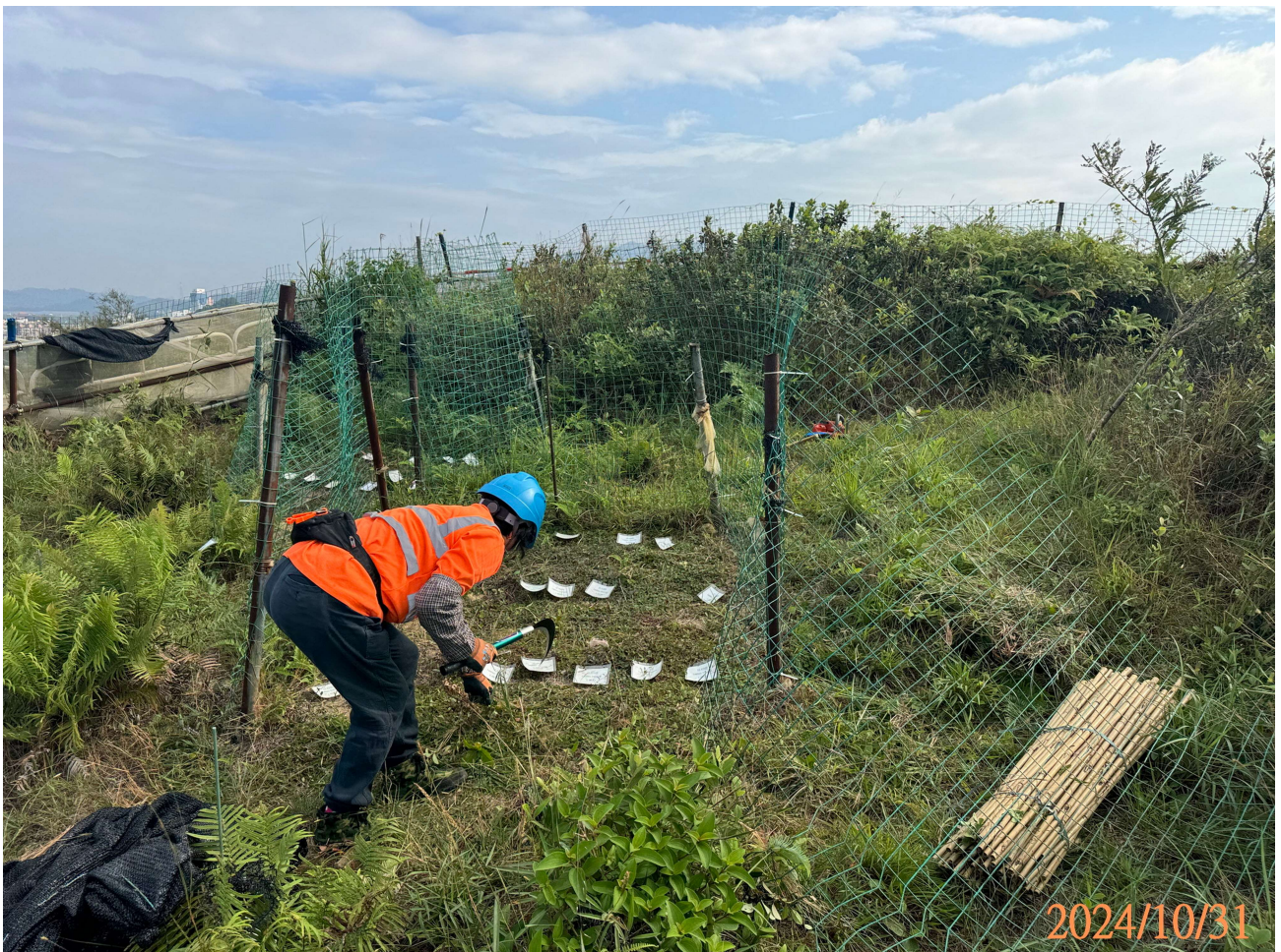
Maintenance works & inspection_2
