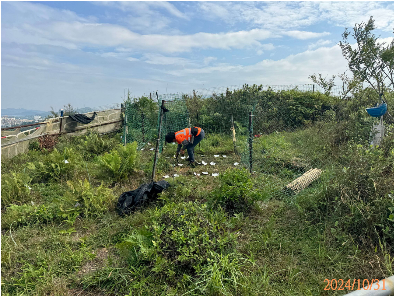
Maintenance works & inspection_1
