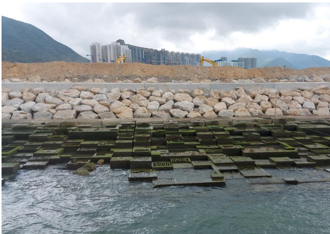
Photo 4 – Natural Rock Material/Planting for Artificial Seawall
