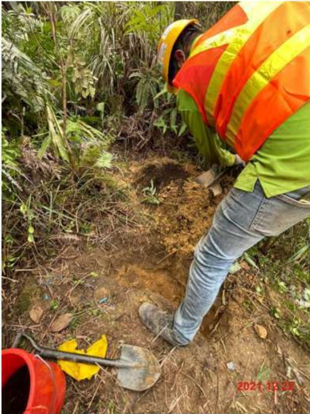
Backfilled with soil mix-A
