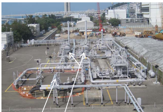
Pipework & Heaters in background
