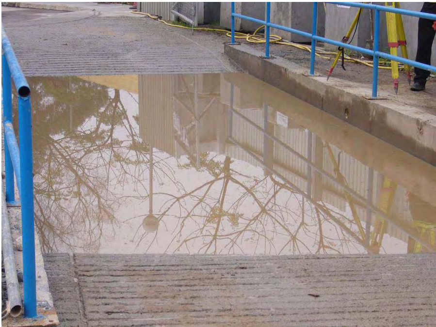
As a reminder, the wheel washing facility should be regularly cleaned up to avoid overflow of muddy water.
