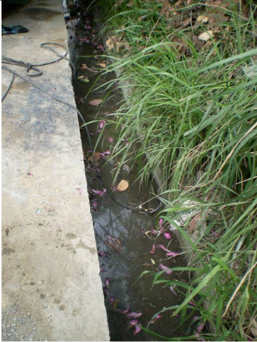
Remark 1: The stagnant water accumulated should be drained away or applied larvidical oil to prevent mosquitoes breeding.
