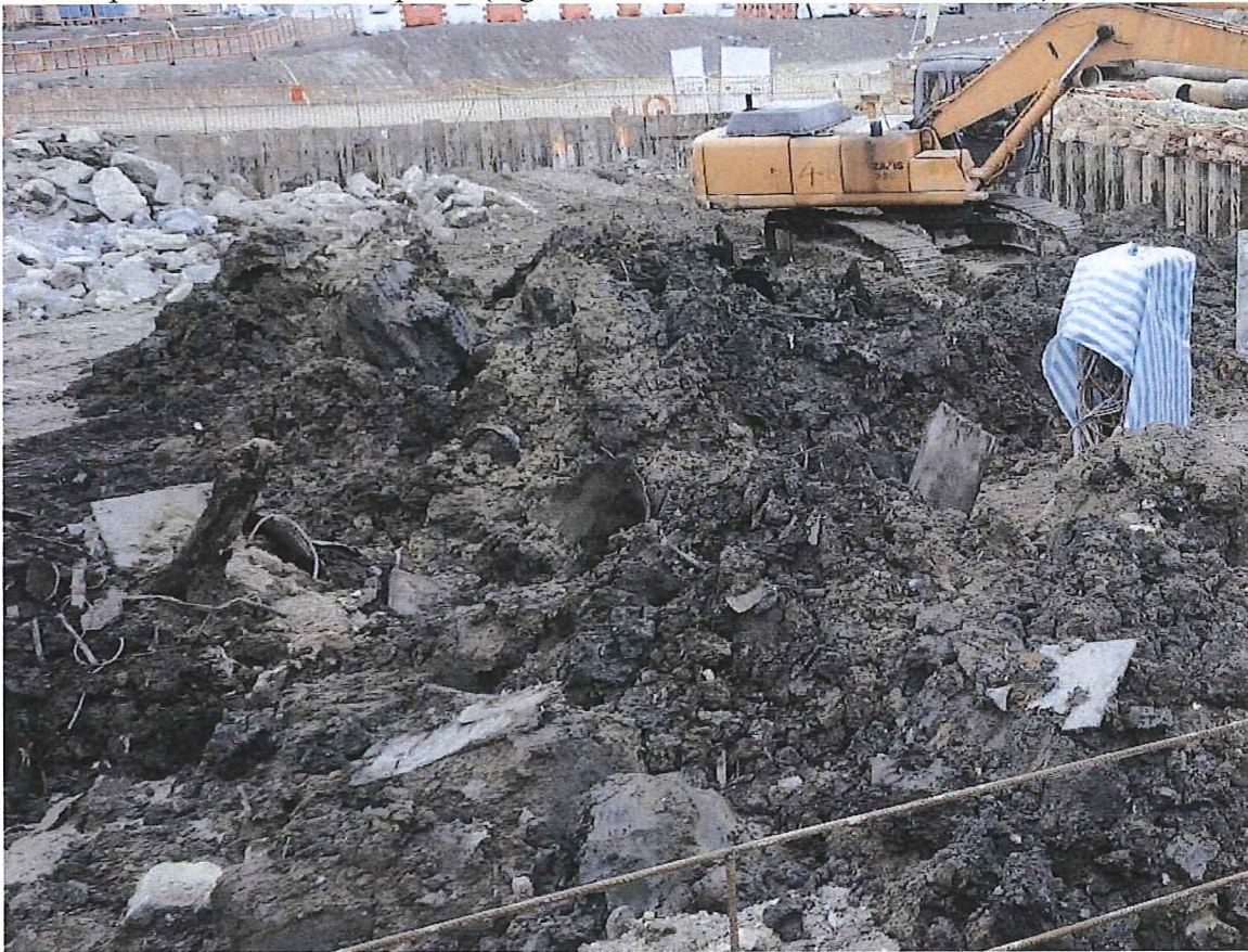
Close-up of the excavated topsoil: (high content of debris and contaminants)
