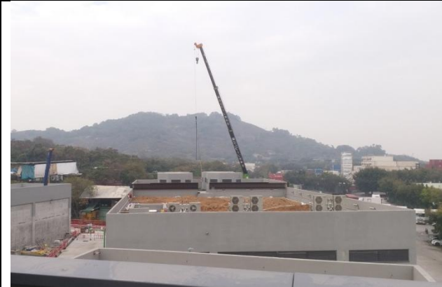
Preparation of the soiling works for green roof at Chemical Building
