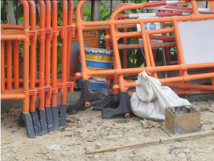
Remark 1: Chemical label and drip tray should be provided for the chemical drum
