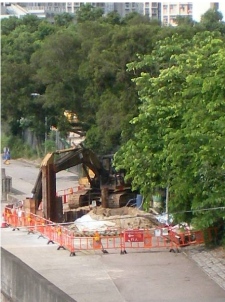
As a general reminder, the stockpile should be covered properly especially on rainy weather to avoid surface runoff.
