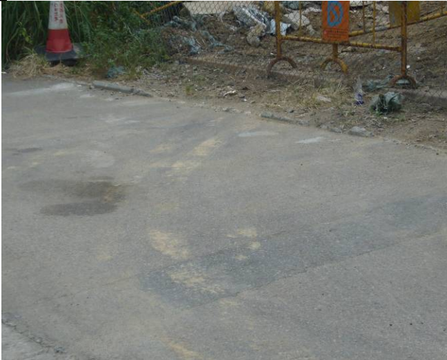
Remark 2: Sand and mud was observed at the public road, the contractor was reminded to clean and keep the public road near the site area was clean.
